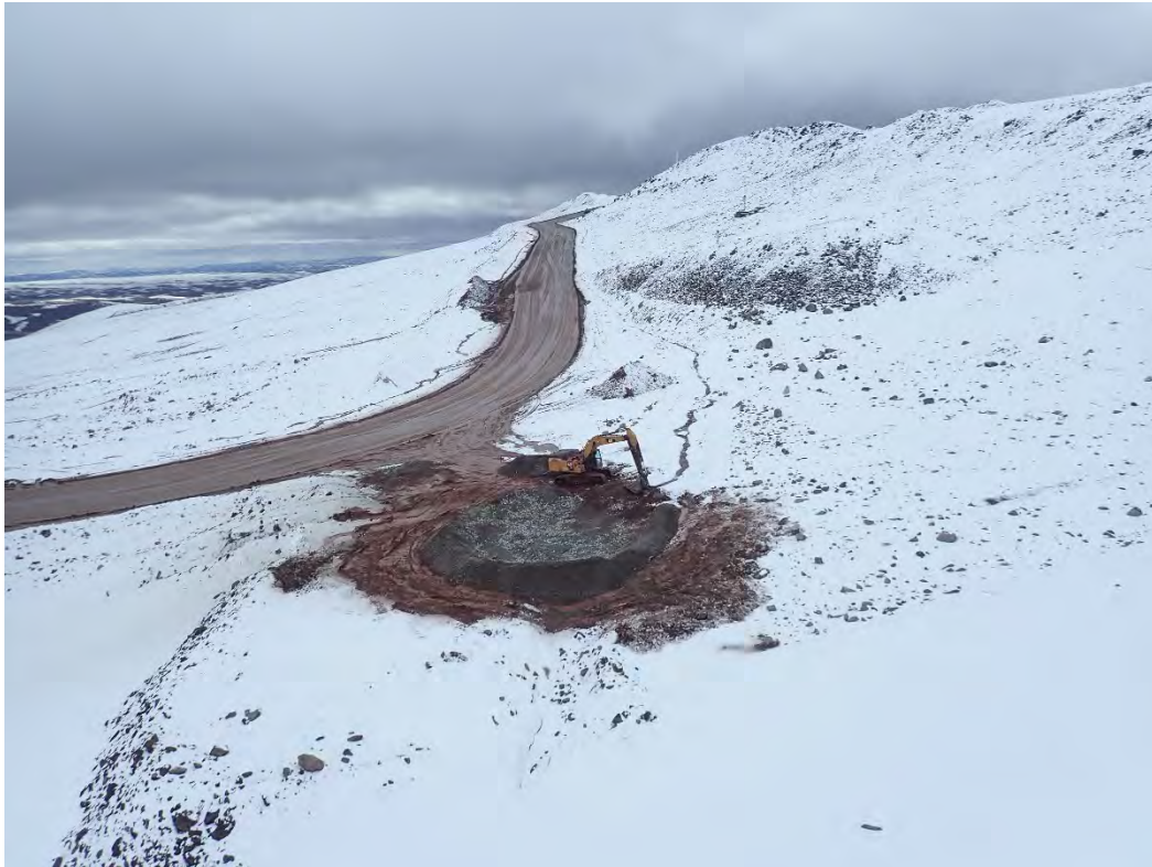
Photo 5. Examples of Sedimentation mitigation measure installation on June 5, 2019
