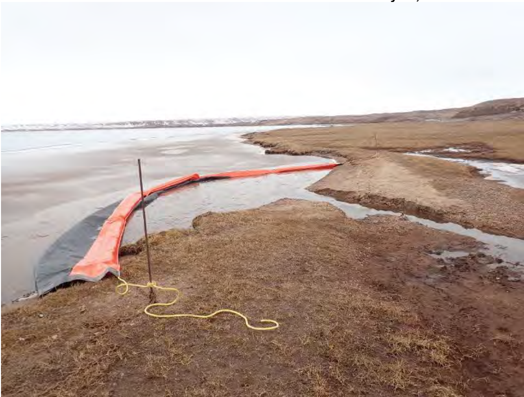
Photo 6. CLSP Outfall into silt curtain on May 10, 2019
