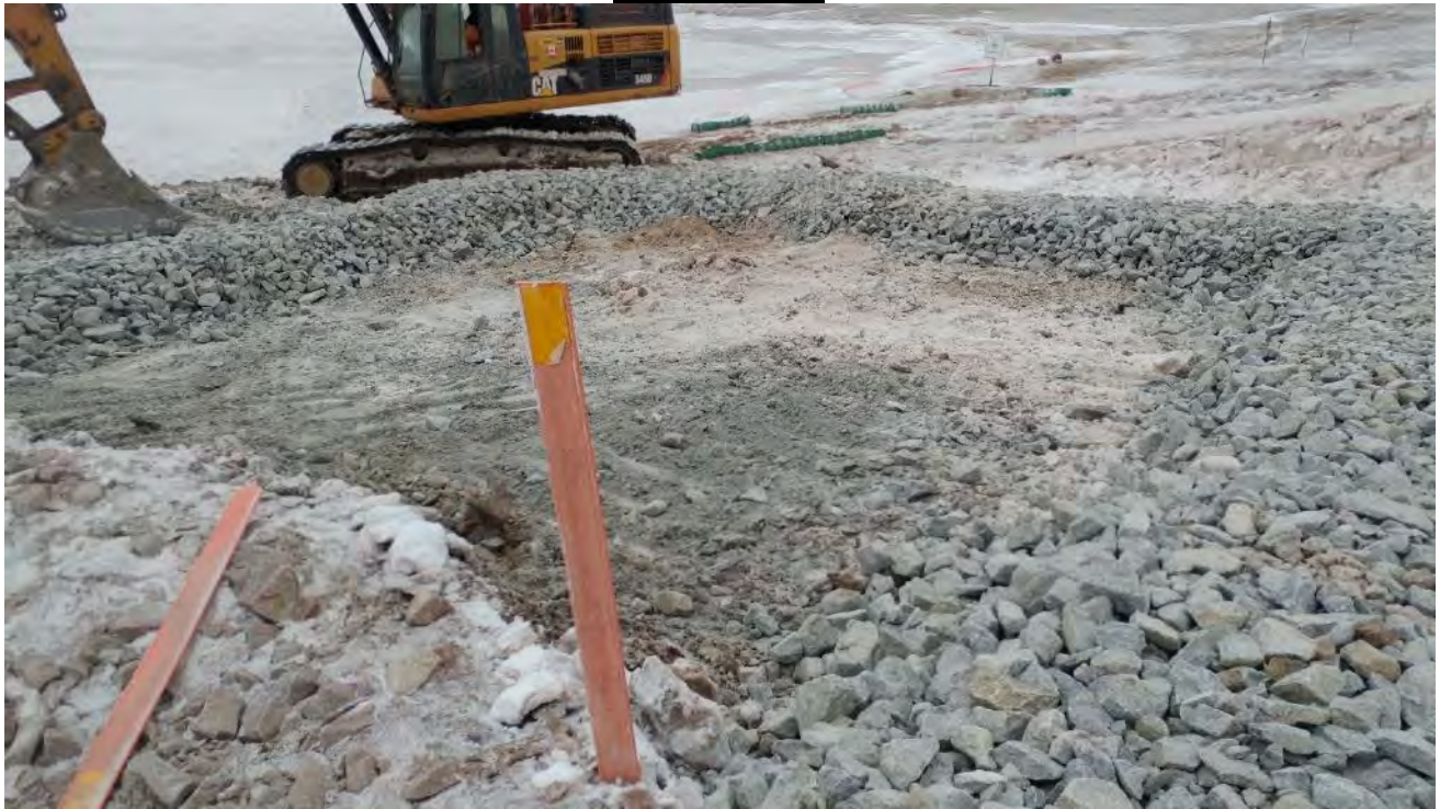
Photo 1. Camp Lake Settling Ponds prior to construction on May 2, 2019
