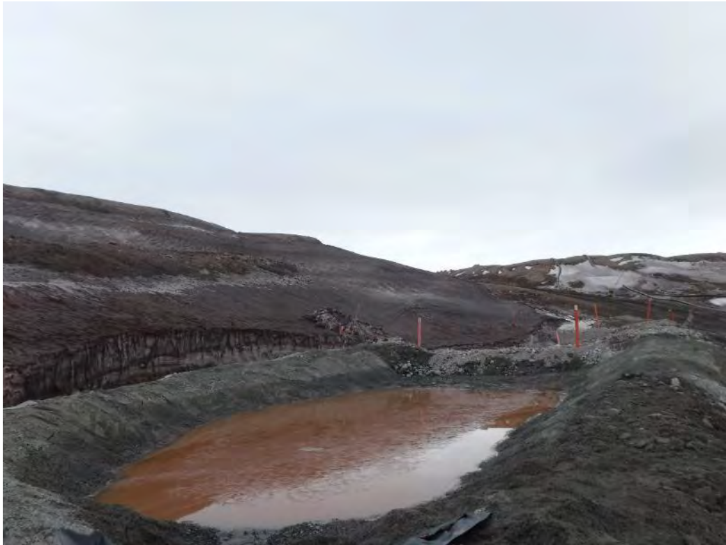
Photo 3. Camp Lake Settling Ponds during construction on May 8, 2019
