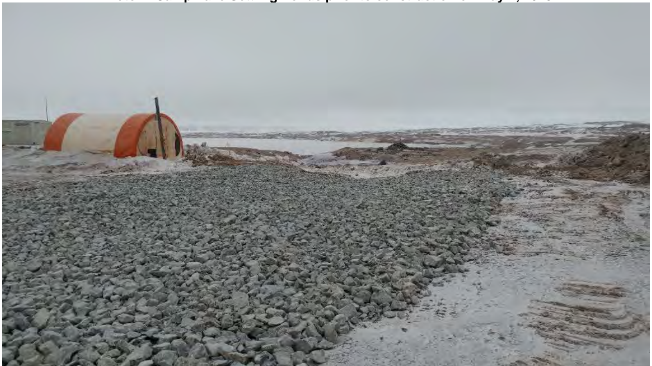
Photo 2. Armouring upstream of the CLSP drainage valley on May 2, 2019
