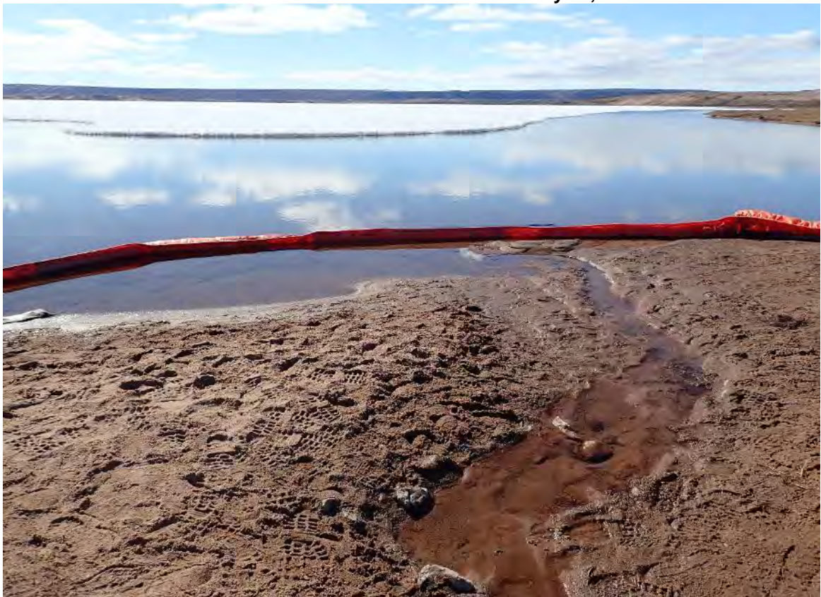
Photo 8. CLSP Outfall on June 6, 2019
