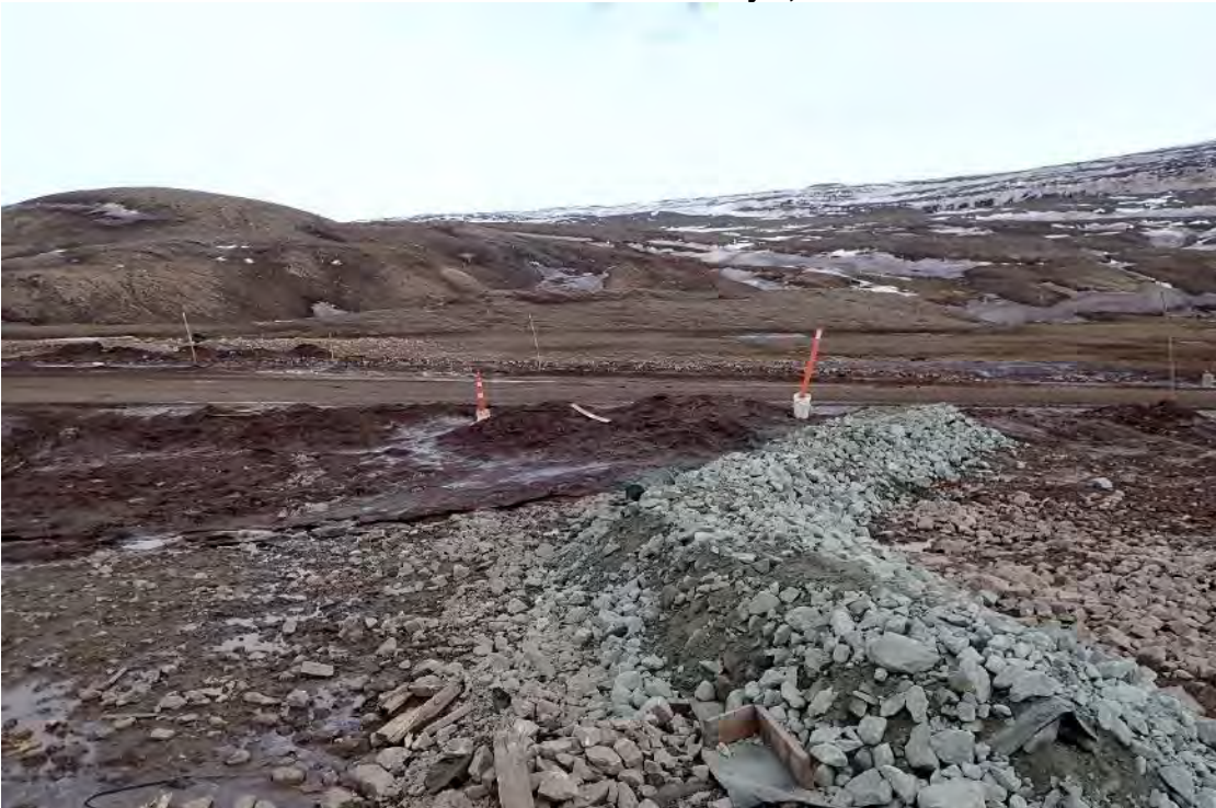
Photo 2. Check dam construction at the outlet of CV-186 on May 8, 2019
