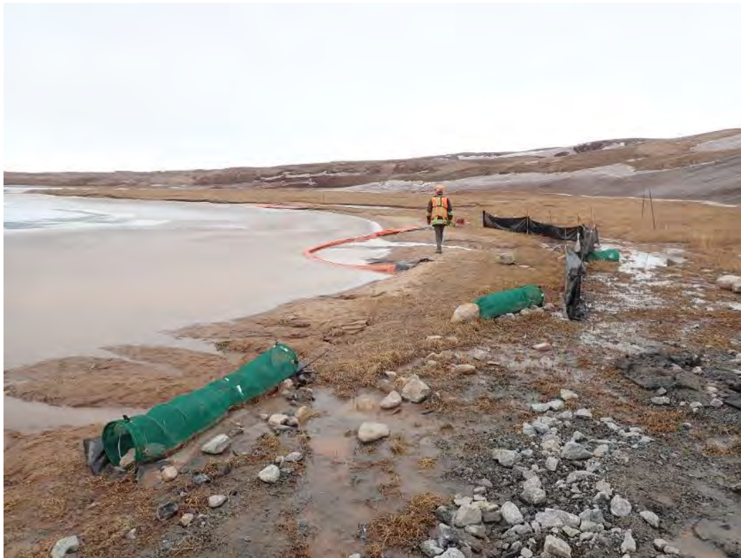
Photo 5. ESC measures at the CLSP Outfall on May 10, 2019
