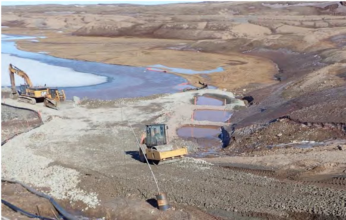
Photo 7. CLSP Outfall construction on May 13, 2019
