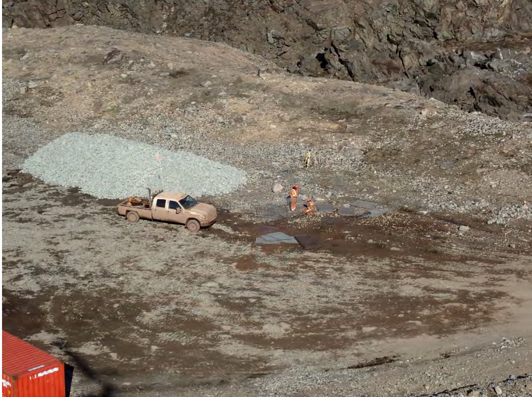
Photo 6. Examples of Sedimentation mitigation measure installation on June 7, 2019
