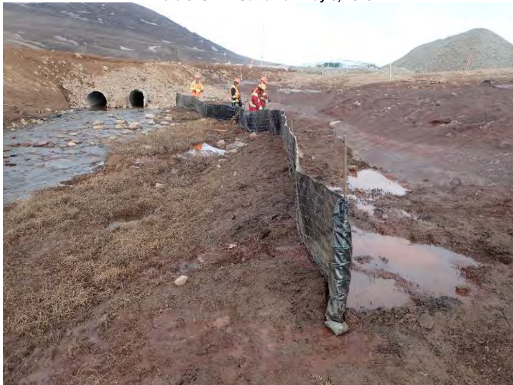
Photo 4. Silt fence installation at the outlet of CV-186 on May 18, 2019
