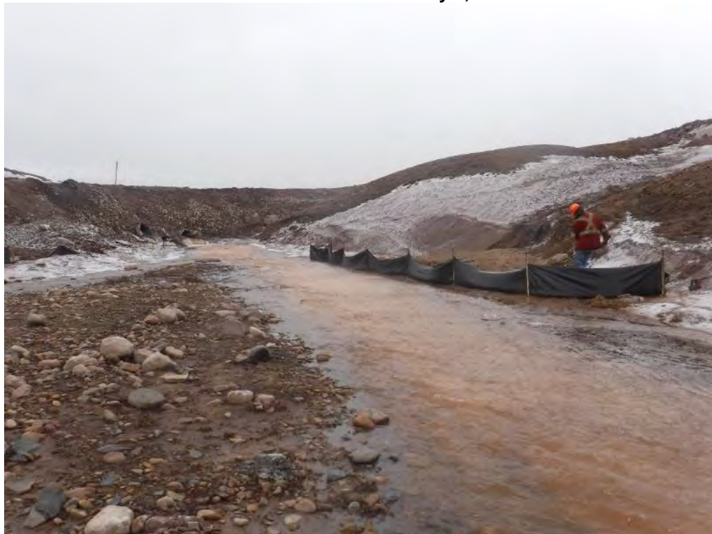
Photo 4. Silt Fencing at the outlet of BG-01 on May 9, 2019
