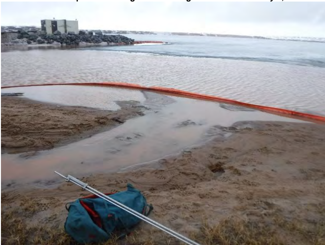
Photo 4. CLSP Outfall into silt curtain on May 9, 2019
