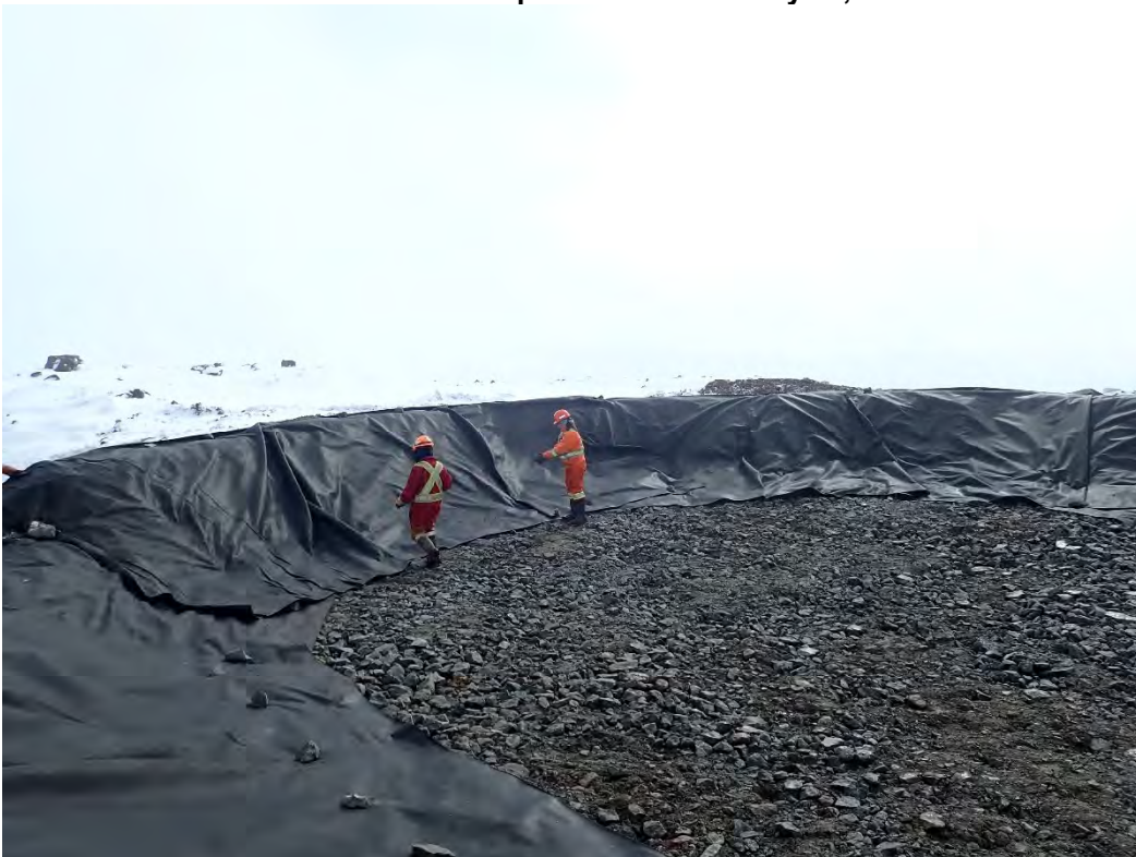
Photo 4. Km 108.5 Check Dam Sedimentation mitigation measure installation on June 5, 2019
