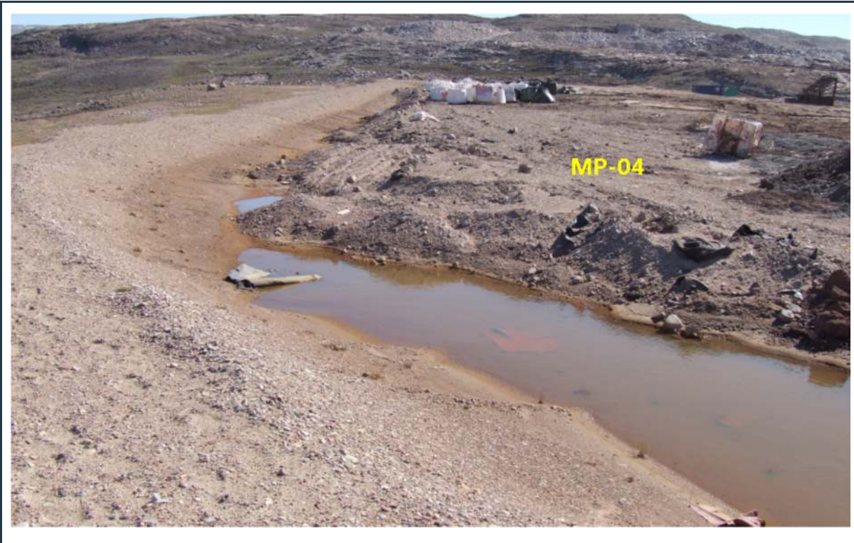
Figure 52: View of the waste and the stable berm at the MP-04 landfarm
