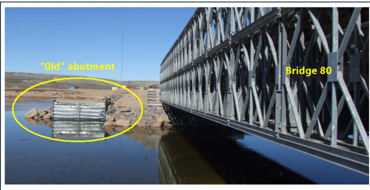
Figure 79: View of bridge 80 with one of the old abutments, looking north
