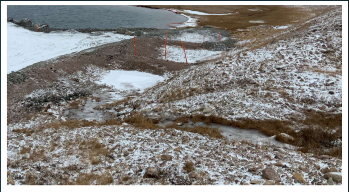
Figure 35: CLSP check berms and silt sedimentation cells.
