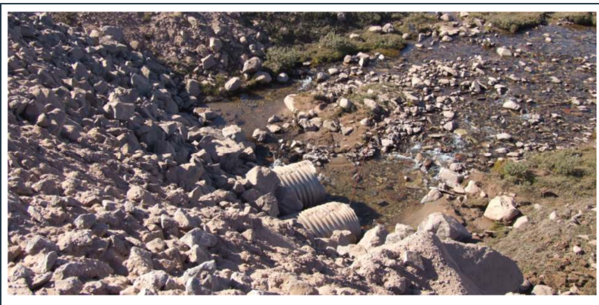
Figure 105: View of culvert 225 (inlet)
