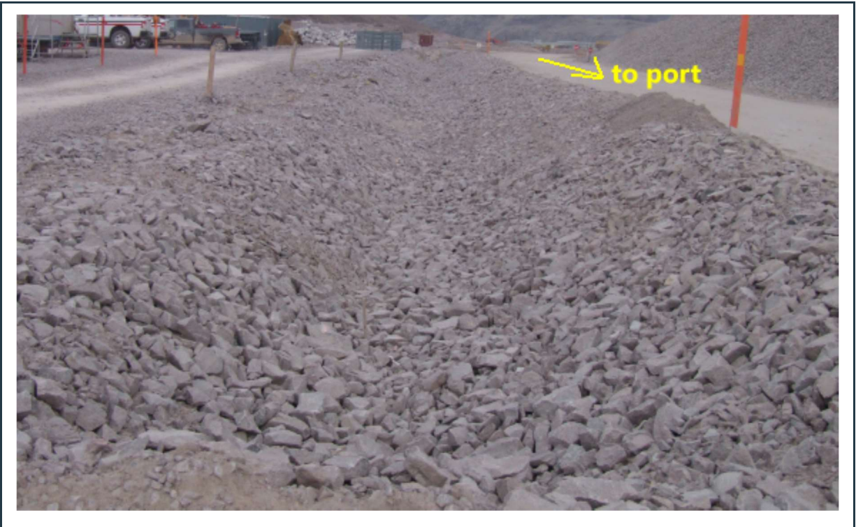
Figure 55: Well maintained "P-SWD-6 Q1 South" surface water collection ditch.
