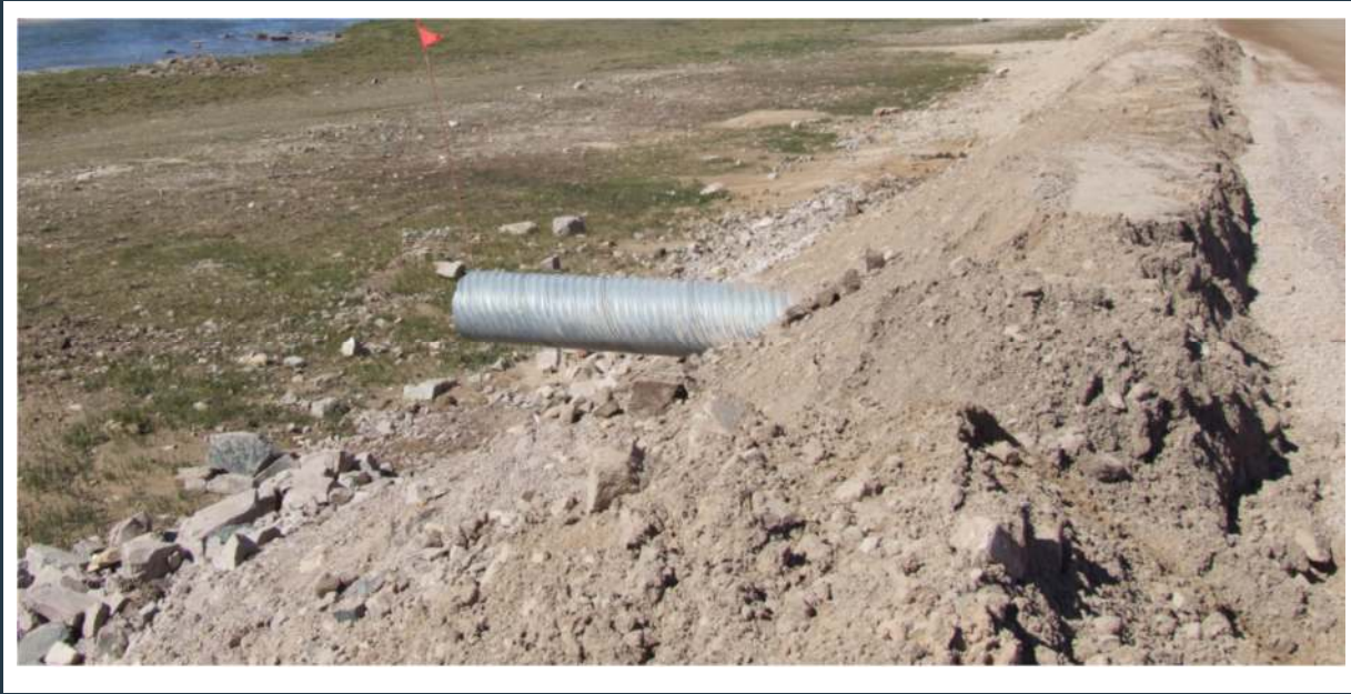
Figure 94: View of culvert 110A (outlet) in good condition
