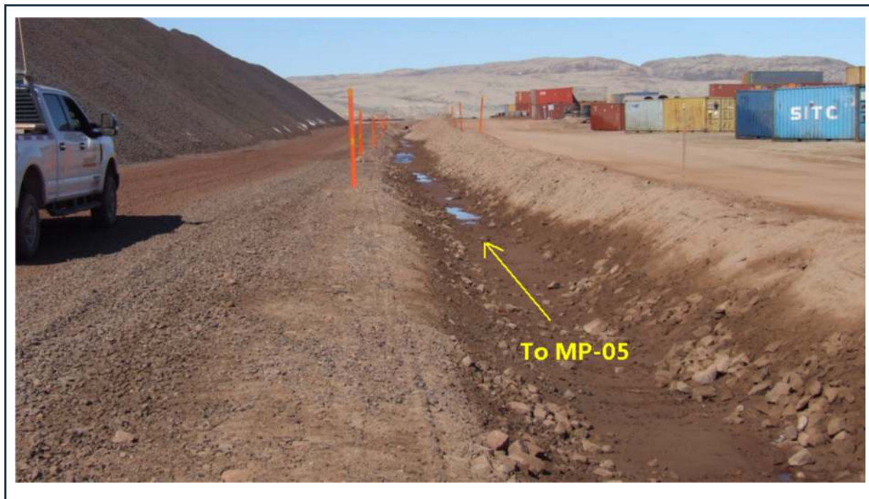
Figure 57: Surface water collection ditch adjacent to stored, crushed ore (leading to the MP-05 pond)
