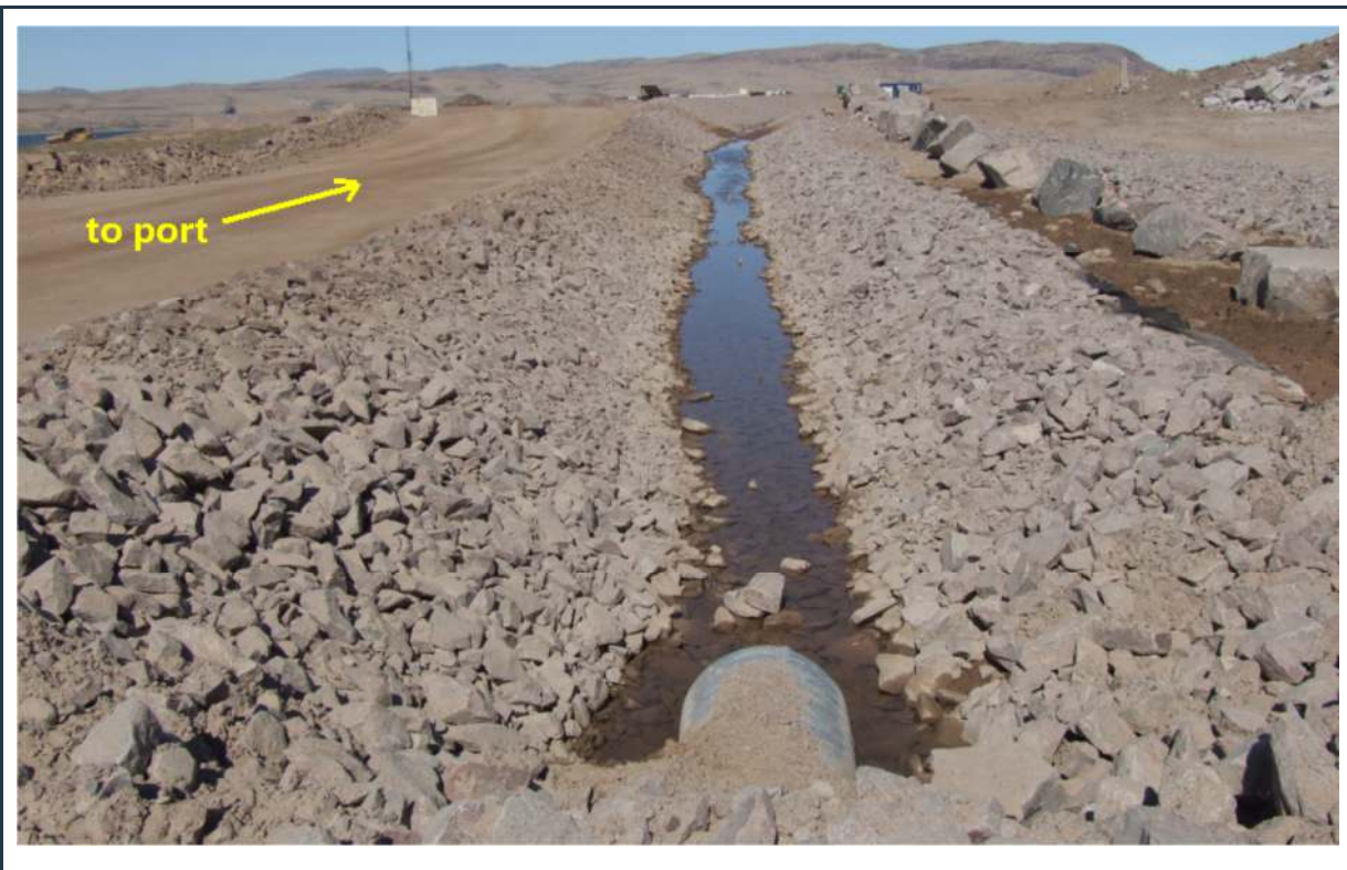
Figure 63: P-SWD-5 Q1 North surface water collection ditch
