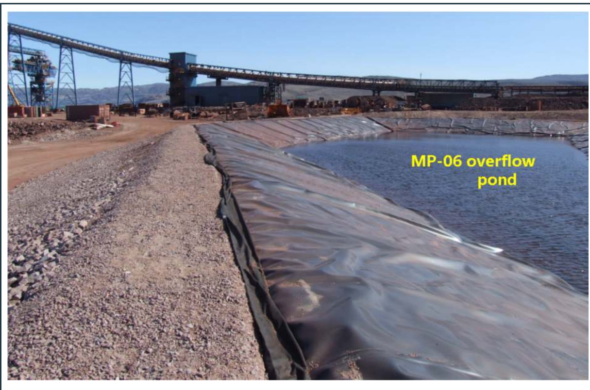
Figure 59: View of the MP-06 overflow pond with stable berm in excellent condition
