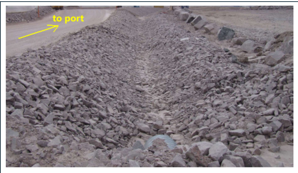
Figure 54: Well maintained "P-SWD-5 Q1 North" surface water collection ditch.
