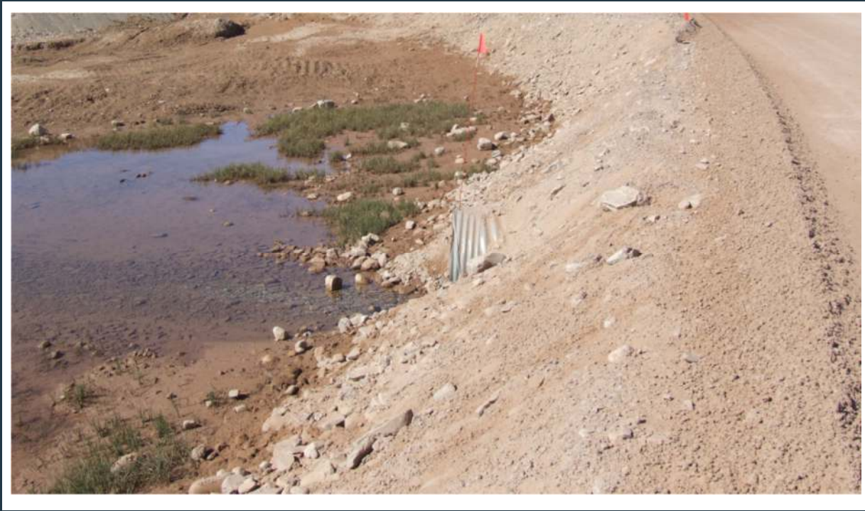
Figure 82: View of culvert 076 (outlet)
