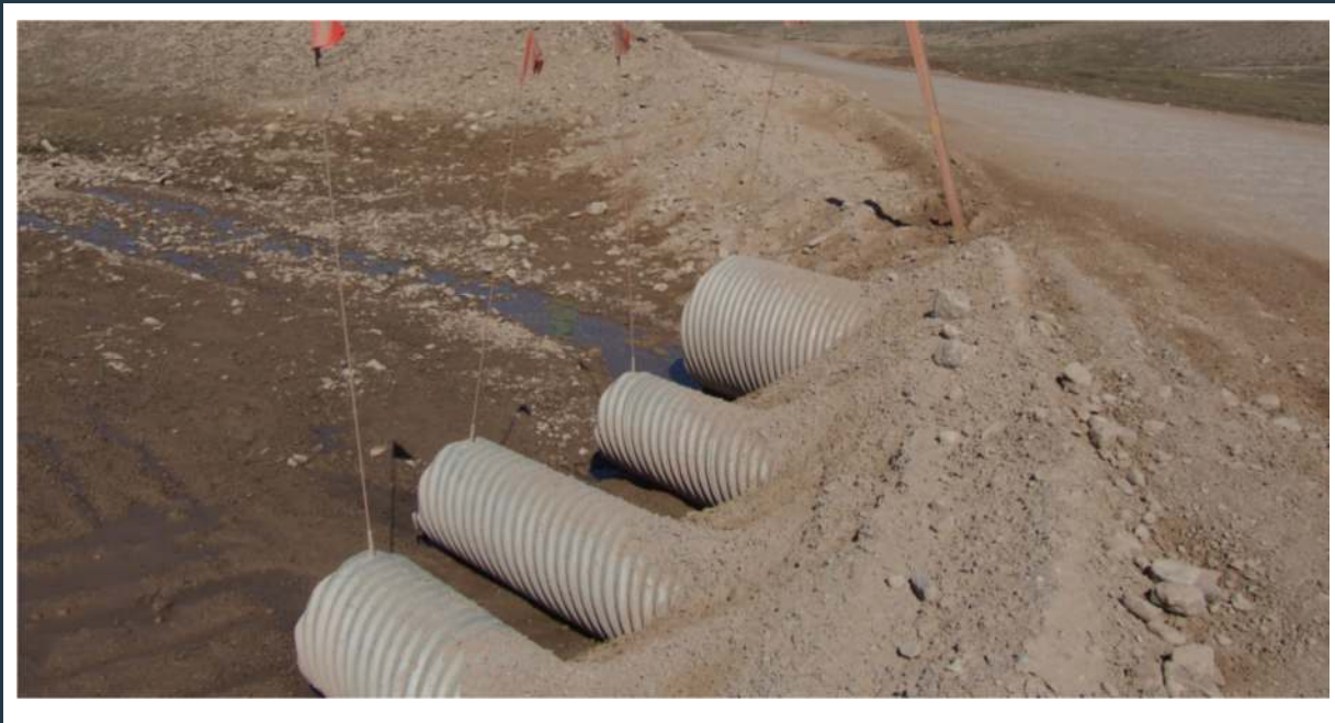
Figure 90: View of culvert(s) 102 (outlet) in excellent conditions
