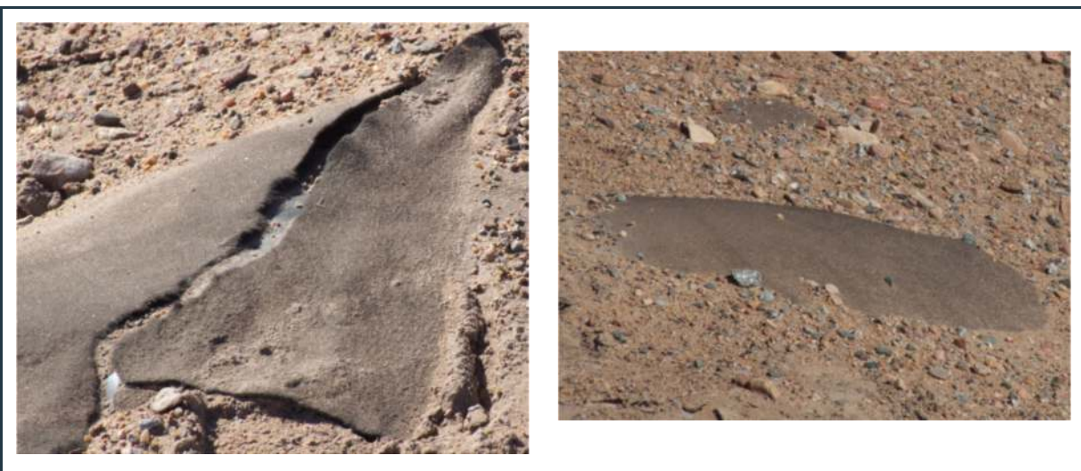
Figure 33: Exposed and ripped geotextile fabric on the berm of the jetfuel farm
