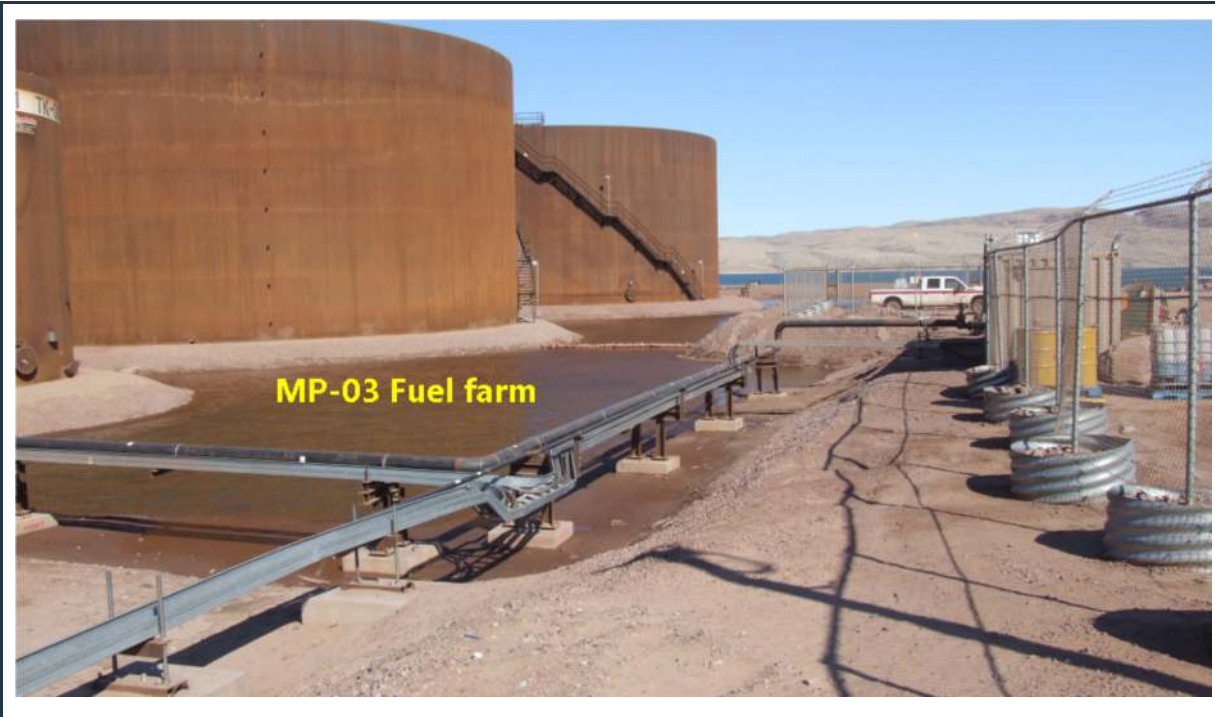
Figure 50: View of stable, well maintained berms around the MP-03 fuel tank farm
