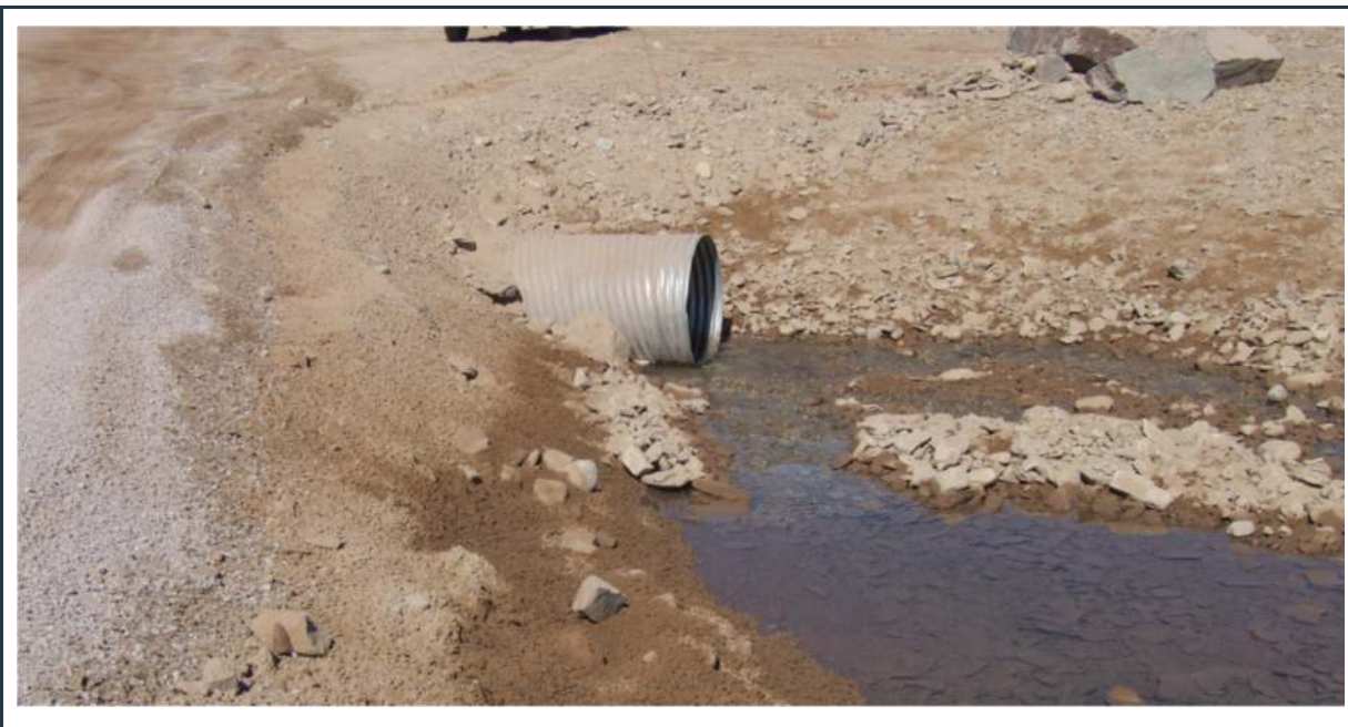
Figure 87: View of culvert 083 (inlet)
