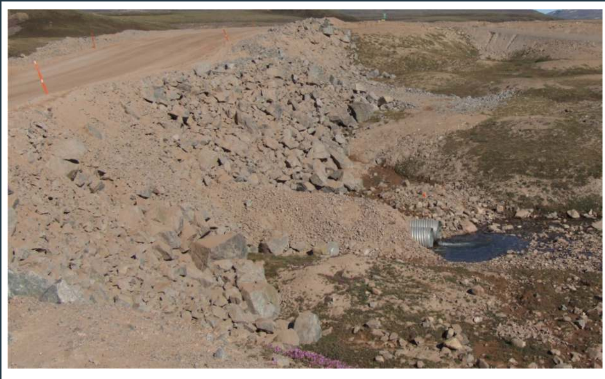
Figure 104: View of culvert 225 (outlet)
