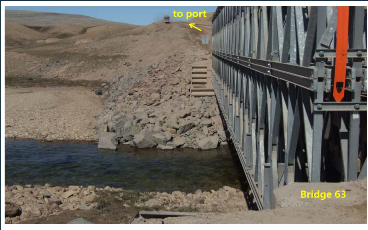
Figure 76: View of bridge 63, looking north
