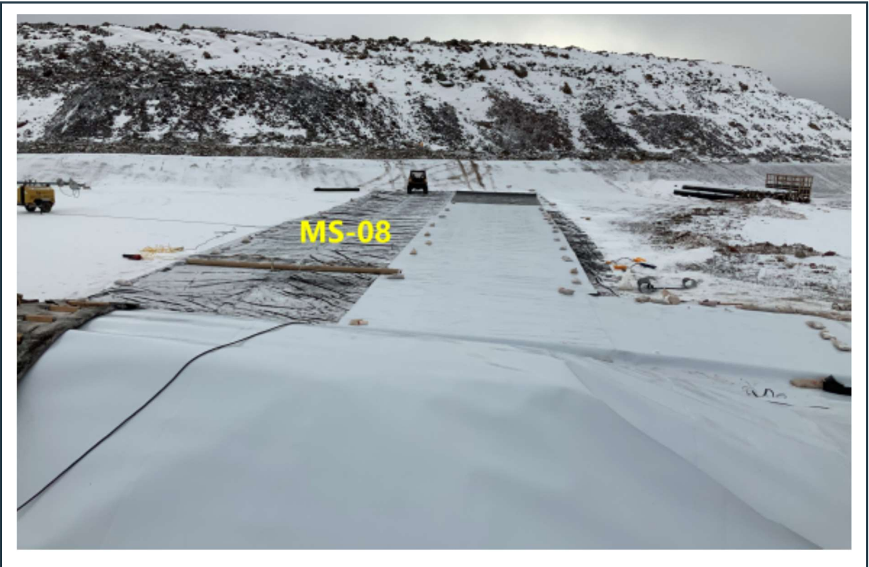
Figure 25: Liner installation in the new MS-08 pond, currently under reconstruction.
