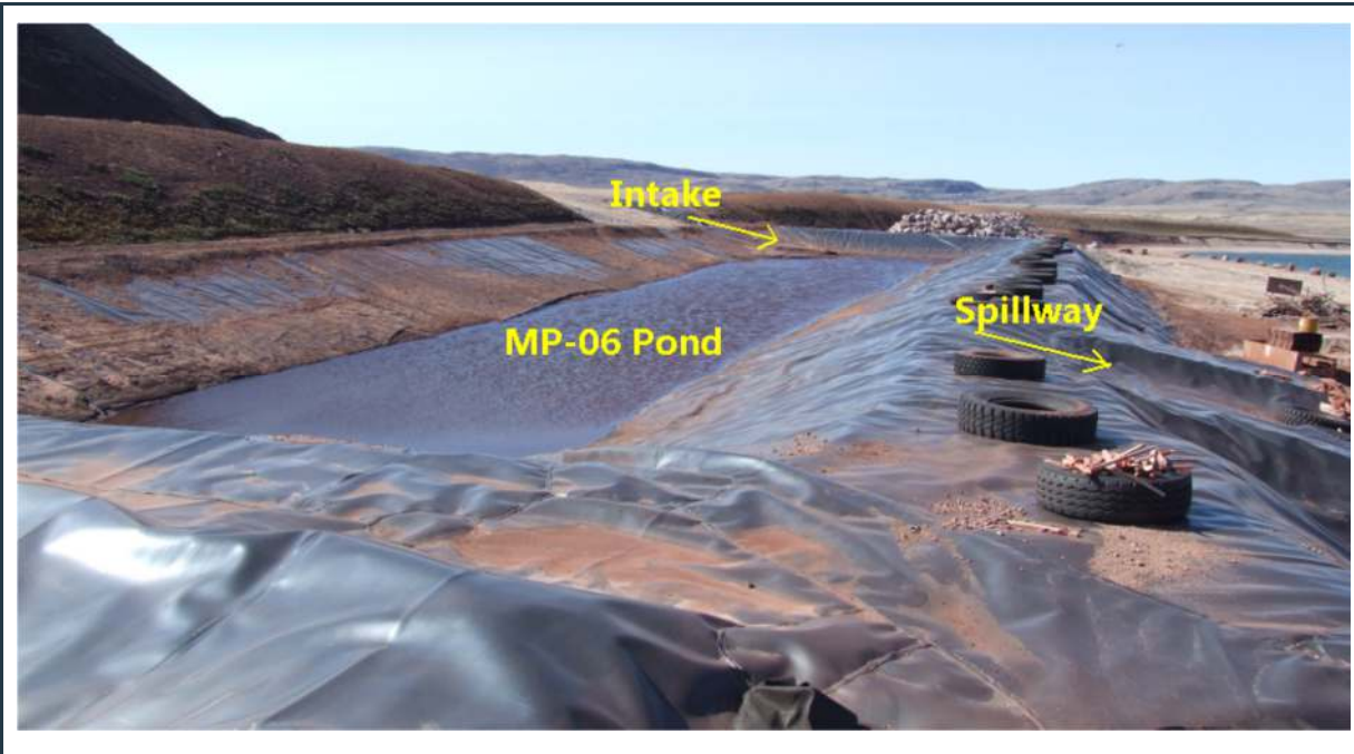
Figure 58: View of the MP-06 pond at the front of the north-west corner of the ore stockpile
