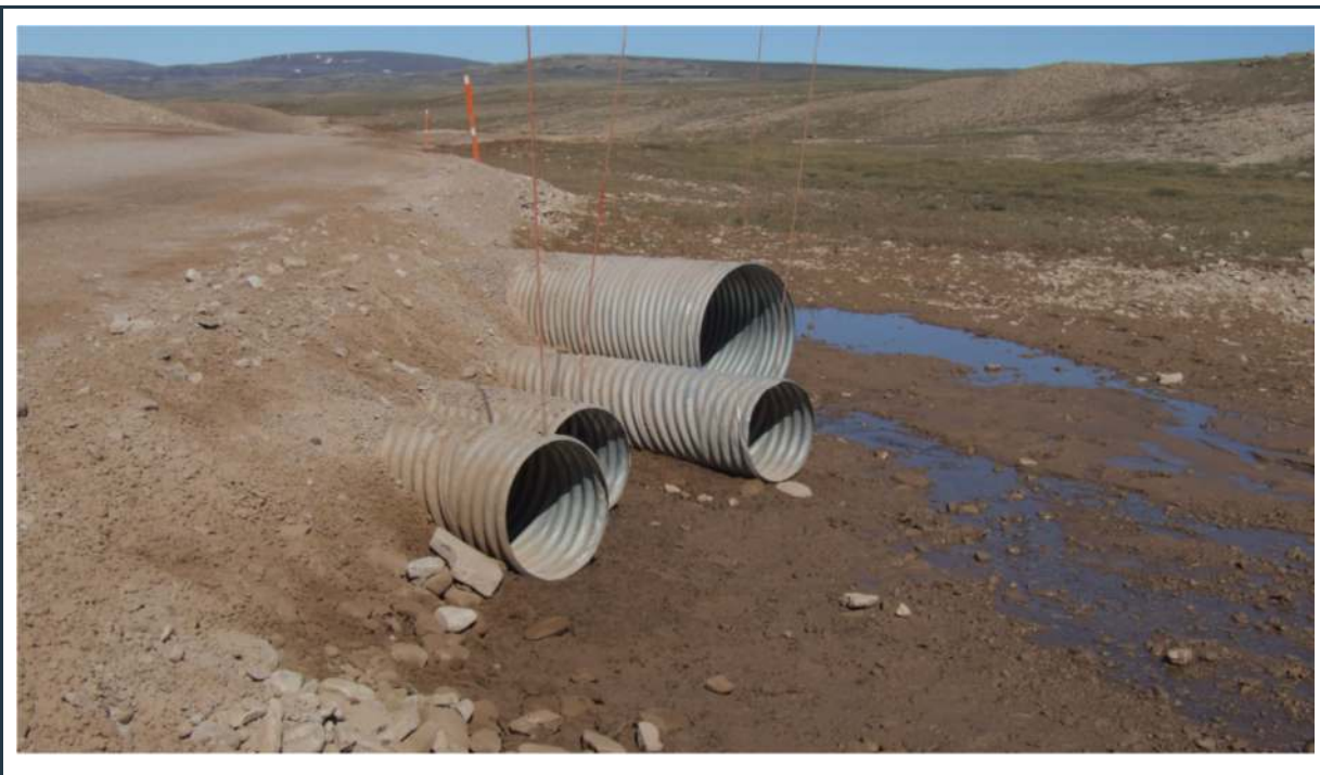
Figure 91: View of culvert(s) 102 (inlet) in excellent conditions
