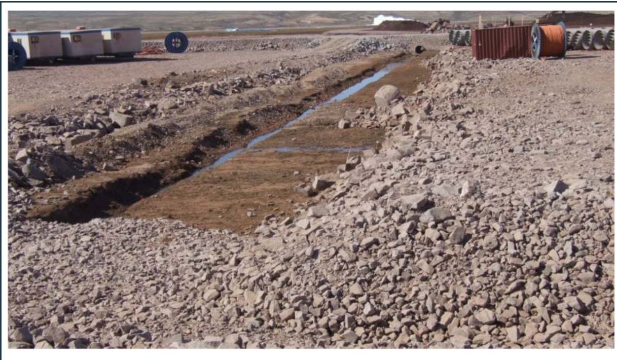
Figure 66: W13-W14 surface water collection ditch (under construction)
