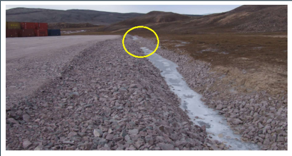
Figure 53: View of the LP2 surface water collection ditch – still under construction.
