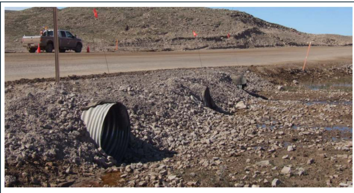
Figure 99: View of culvert(s) 112D (inlet)
