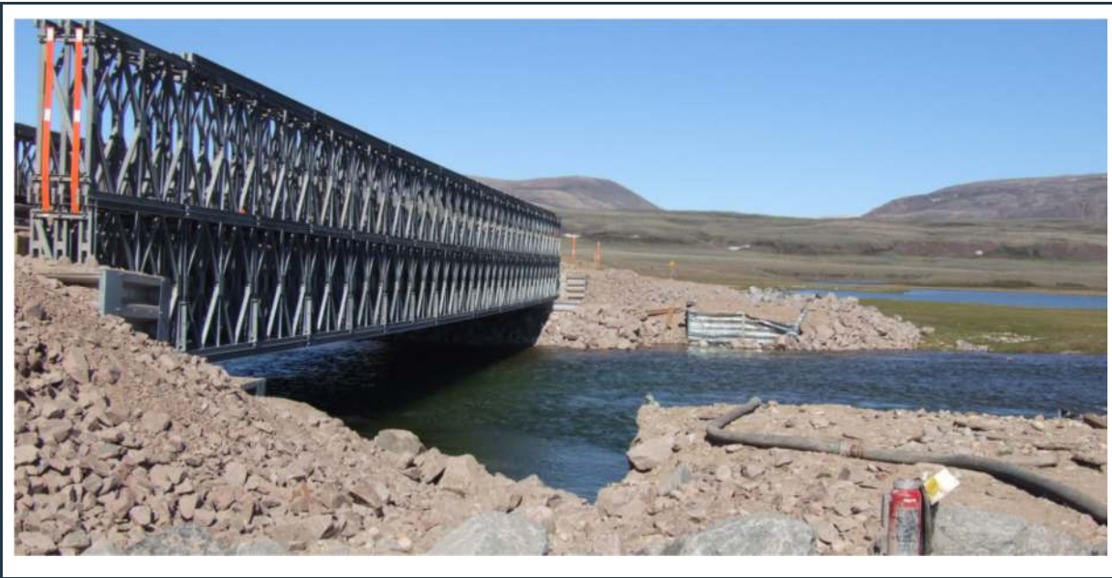
Figure 72: View of bridge 17 (17 km from the port), looking north-east
