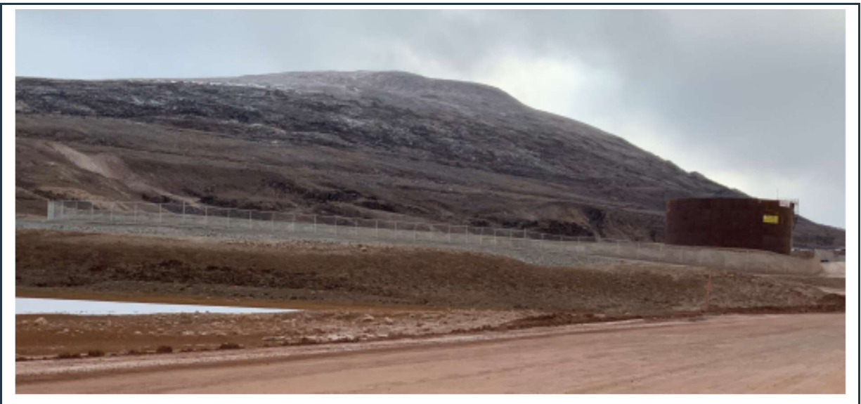
Figure 32: View of the recently completed new fuel storage.
