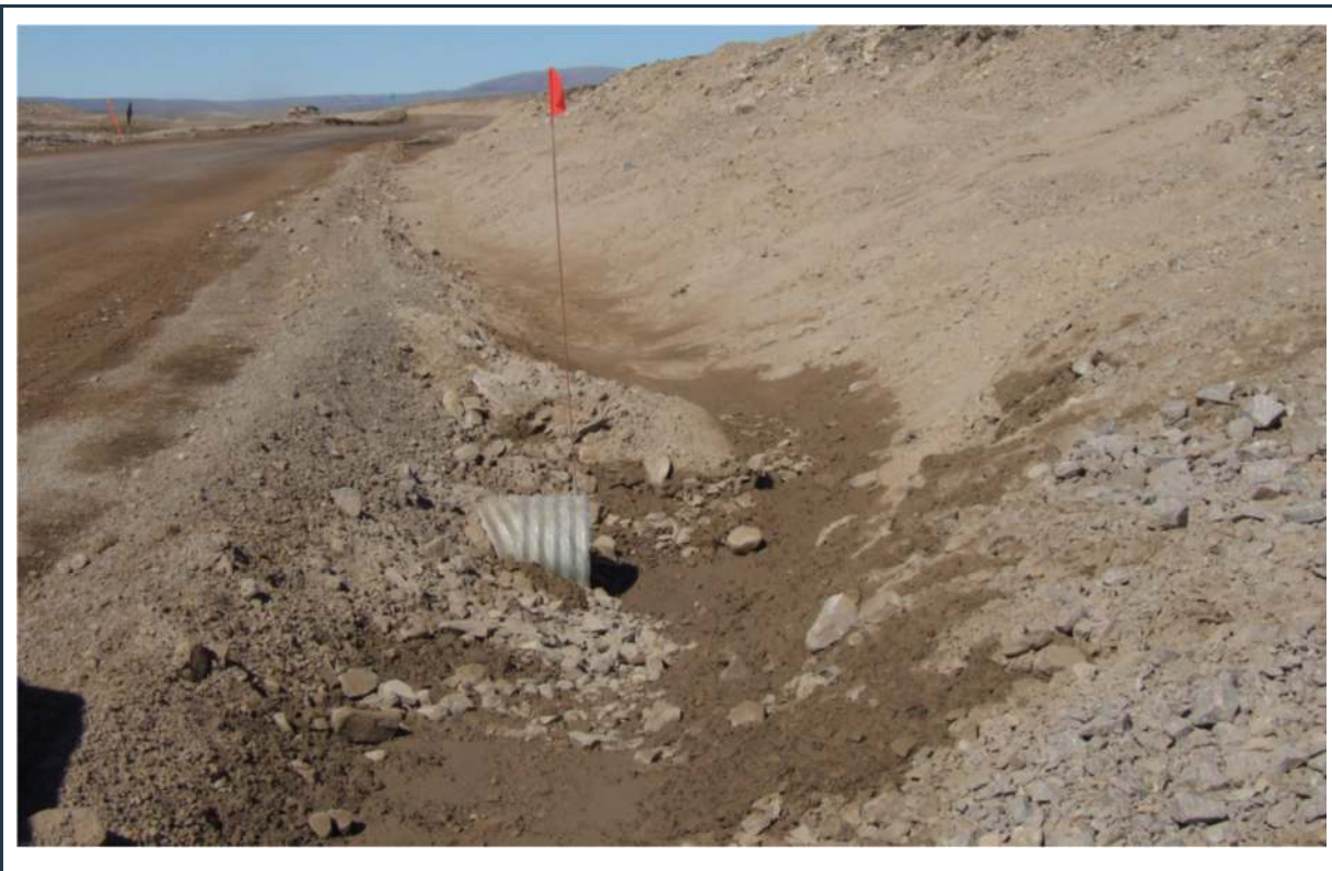
Figure 95: View of culvert 110A (inlet) in good condition
