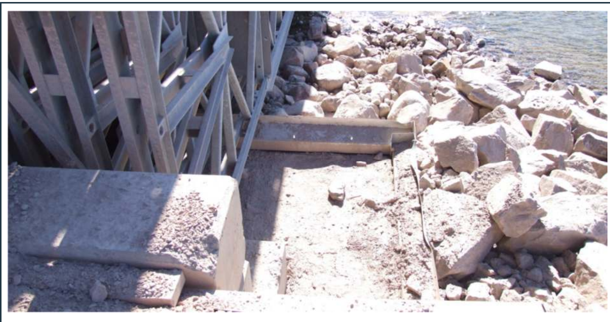
Figure 73: Foundation and rip-rap conditions at one of the abutments at bridge 17
