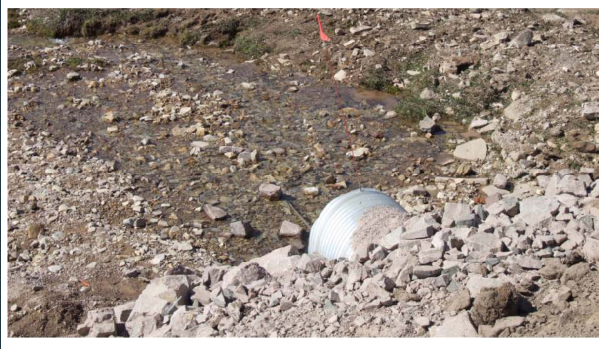
Figure 96: View of culvert 111 (outlet)
