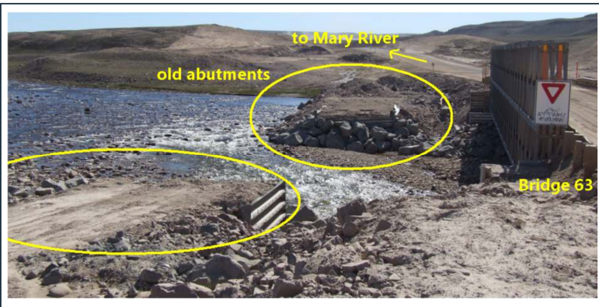
Figure 77: View of the "old" abutments at bridge 63
