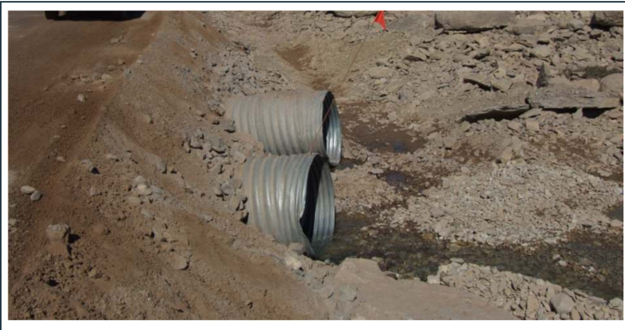
Figure 89: View of culvert(s) 094 (inlet) in excellent conditions
