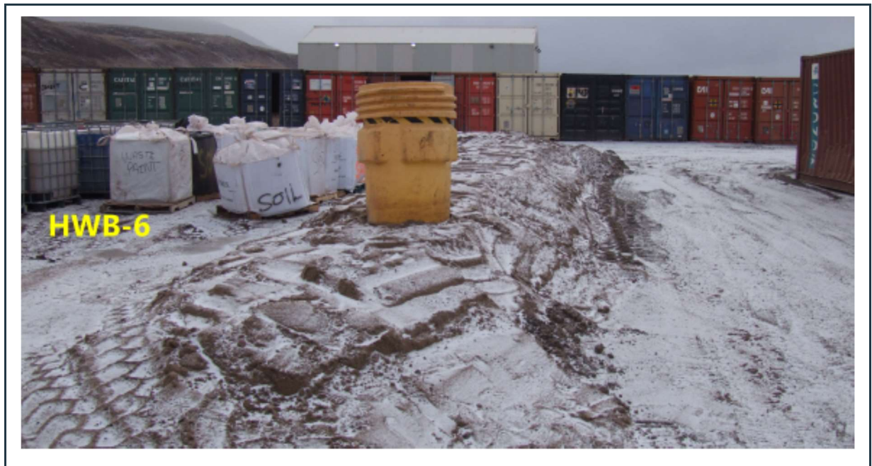
Figure 14: View of the HWB-6 cell, with additional fill placed recently on the berm.
