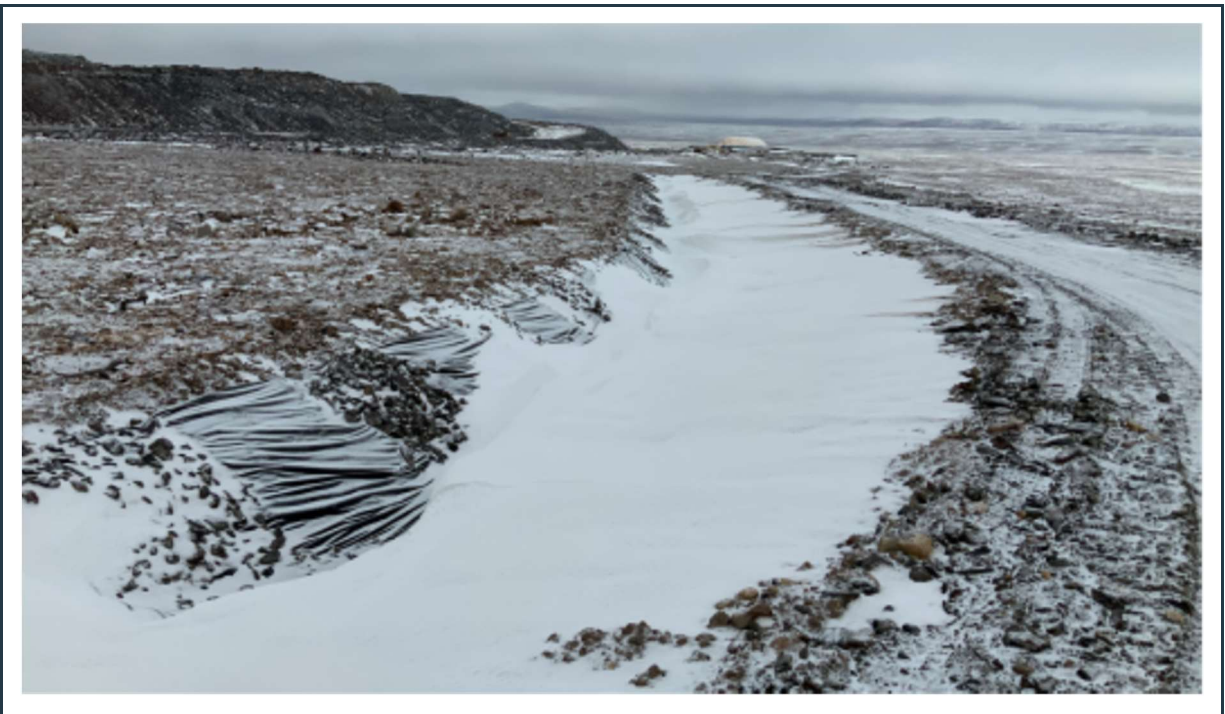
Figure 22: Snow-filled ditch under construction around the waste rock dump (south-east side).
