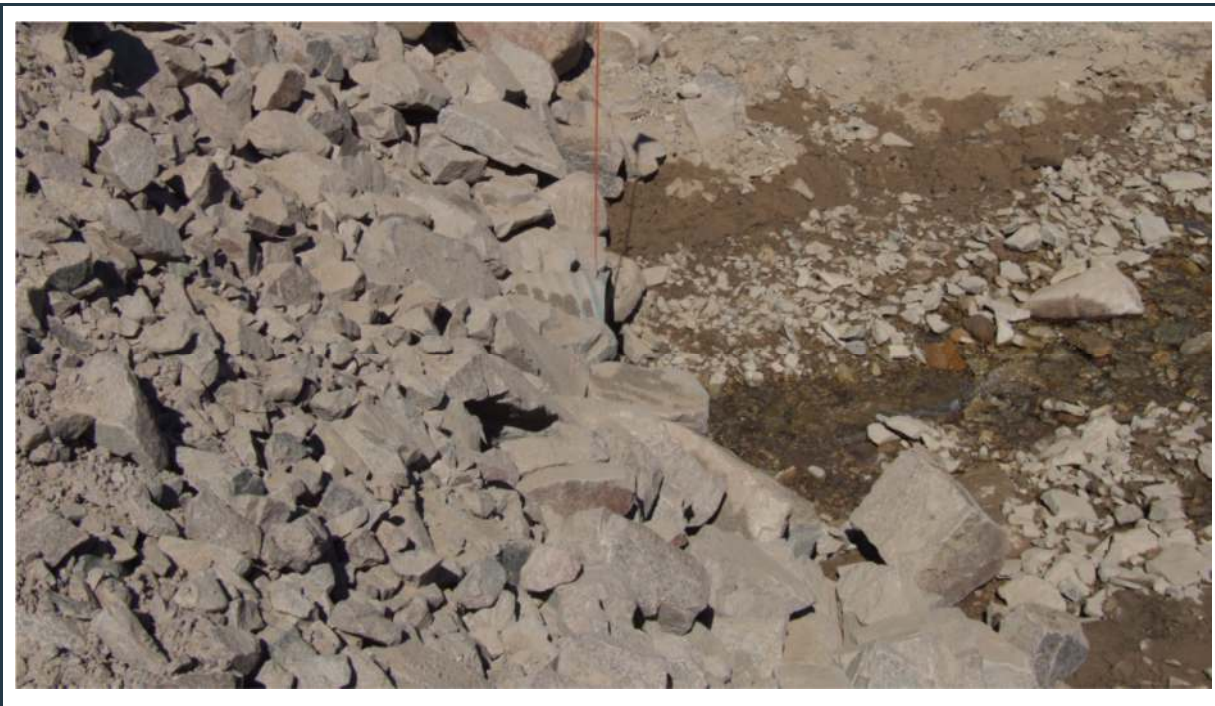
Figure 97: View of culvert 111 (inlet)
