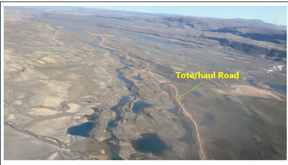
Figure 5: Section of the tote/haul road between the Mary River Mine site and Milne Inlet Port
