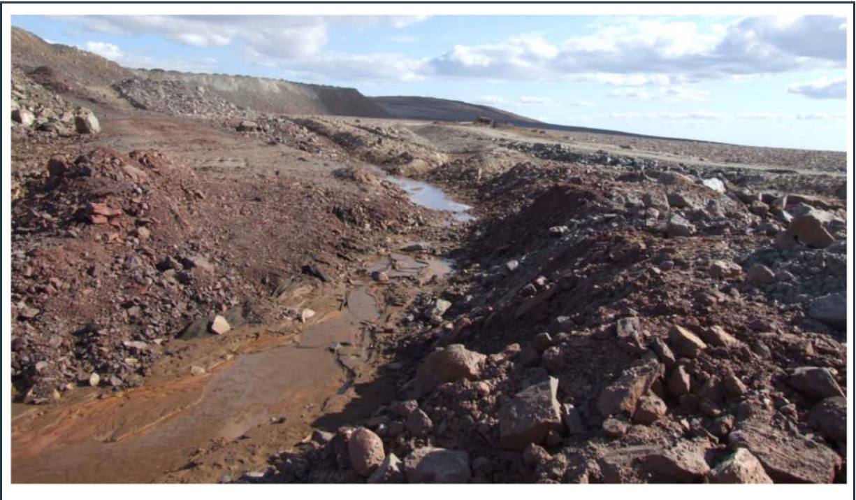
Figure 26: Side-ditch under construction around the waste rock dump
