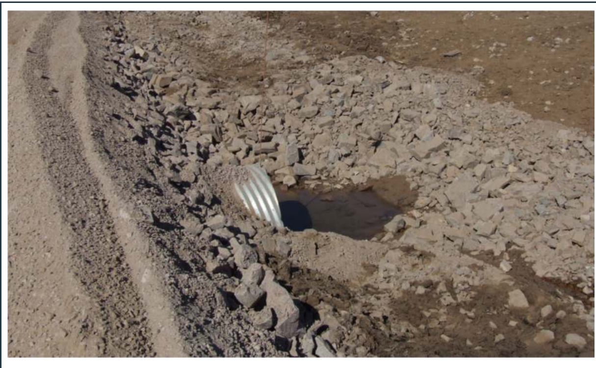
Figure 103: View of culvert 202 (inlet)
