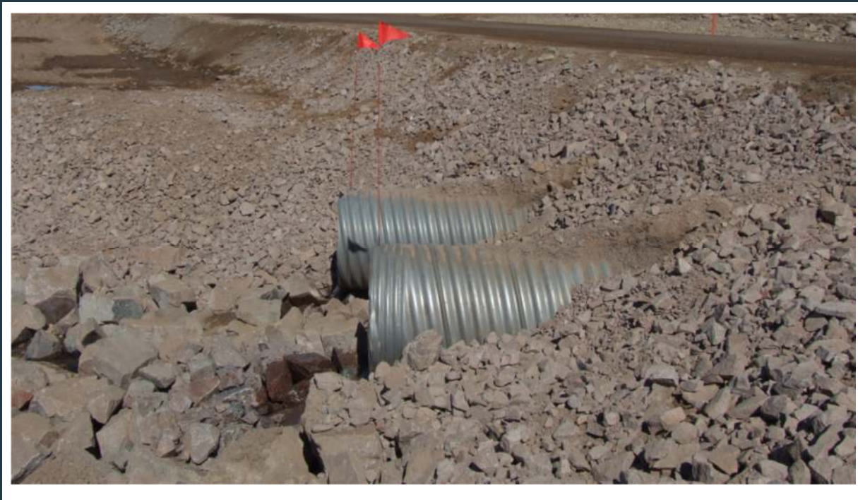
Figure 88: View of culvert(s) 094 (outlet) in excellent conditions
