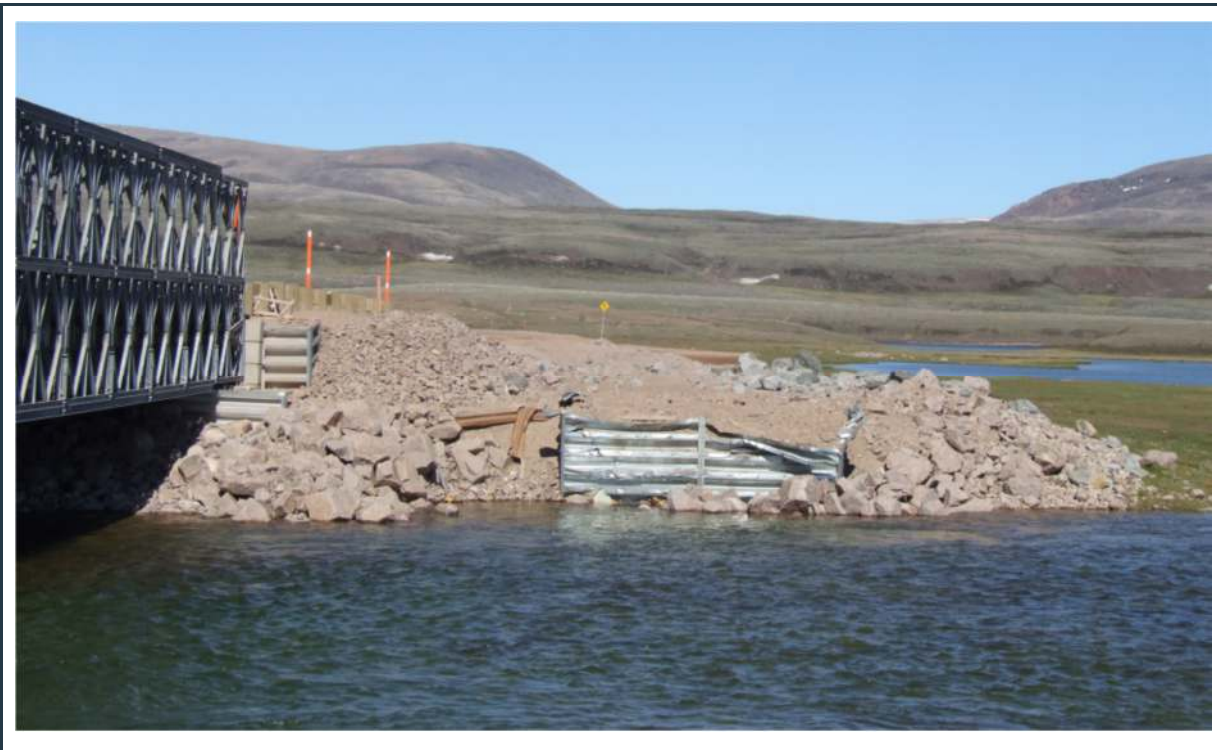
Figure 75: The “old” north-east abutment at bridge 17
