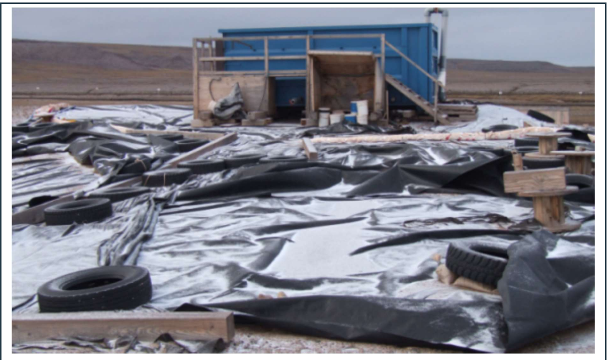
Figure 8: PWSP #2 and #3 – Untidy conditions at the water discharge point between ponds #2 and #3.
