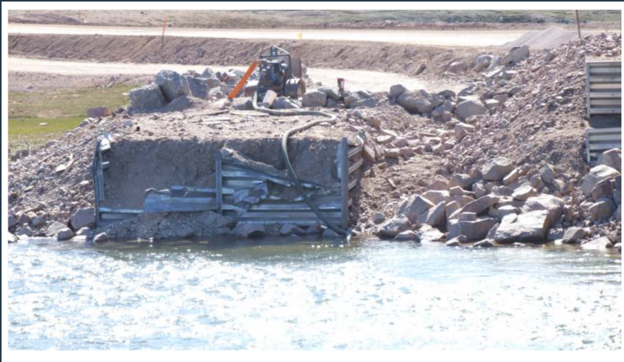
Figure 74: The “old” south-east abutment at bridge 17
