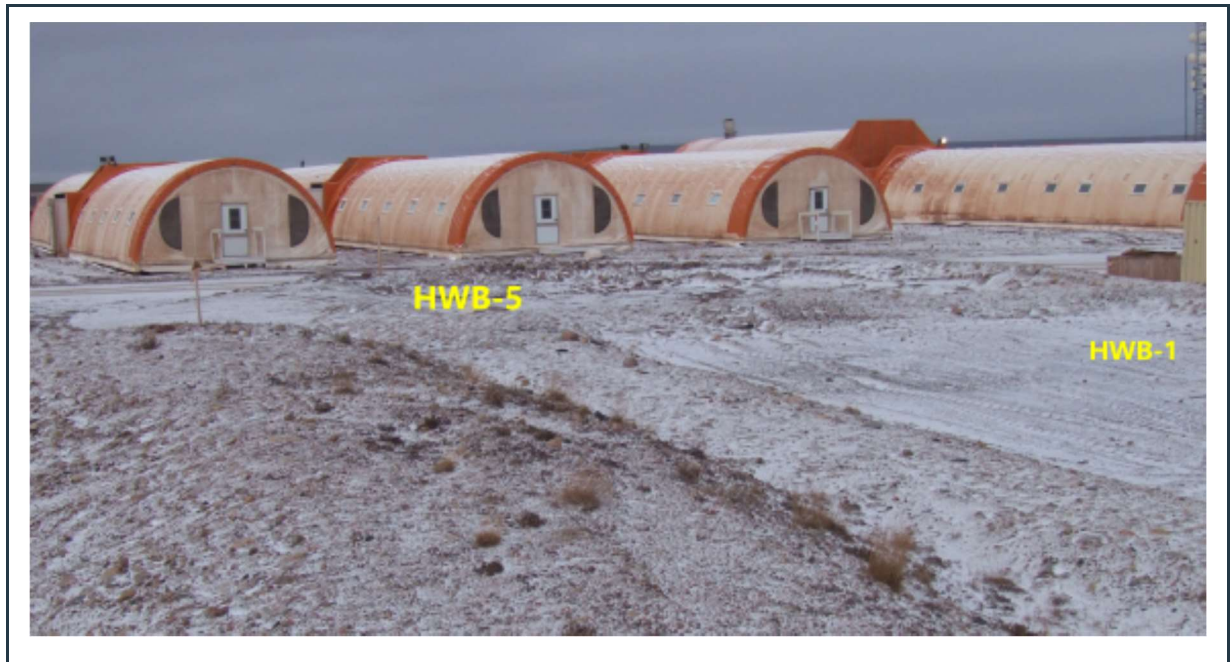
Figure 13: View of HWB-5, located immediately adjacent to HWB-1. Both cells are currently empty.
