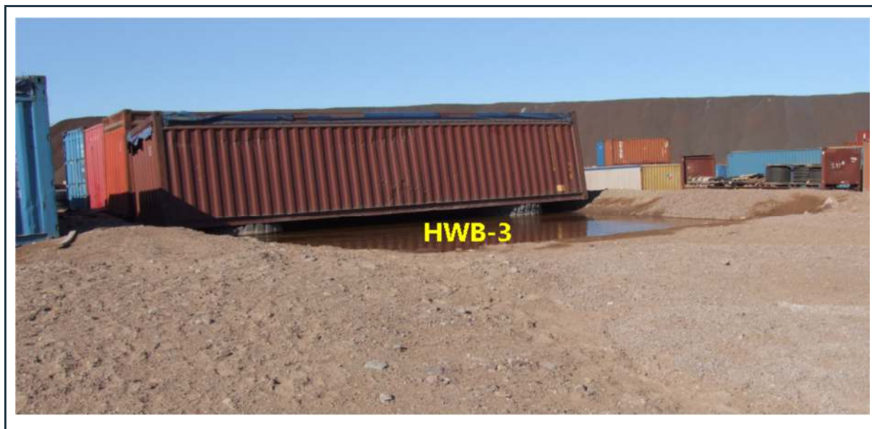
Figure 45: View of the HWB-3 cell, containing shipping containers
