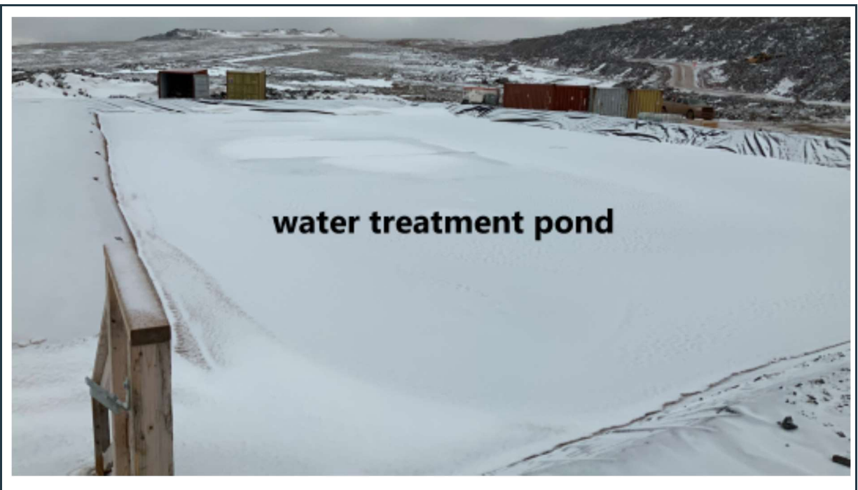
Figure 26: Water treatment pond adjacent to the waste rock dump and MS-08 (ice and snow covered).
