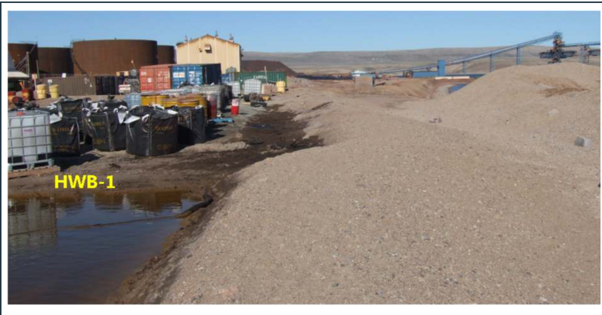
Figure 42: View of the HWB-1 pond with stable berm and ponding water within the cell
