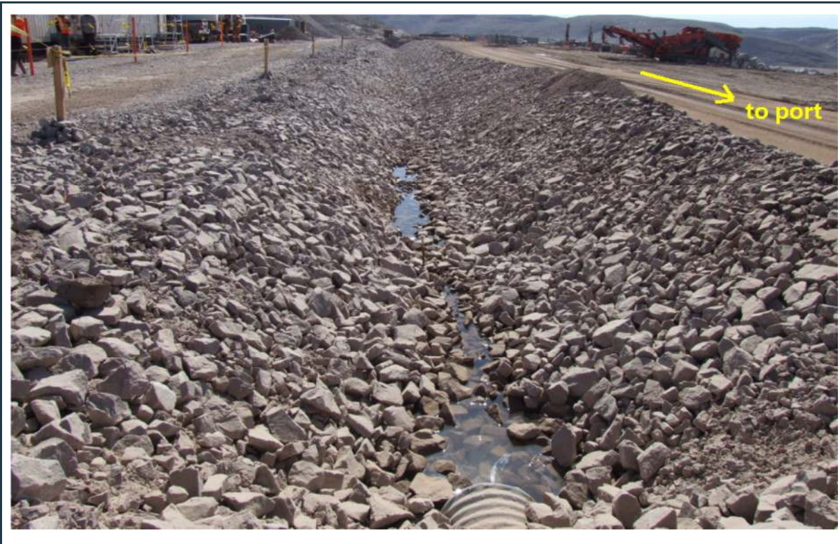
Figure 64: P-SWD-6 Q1 South surface water collection ditch
