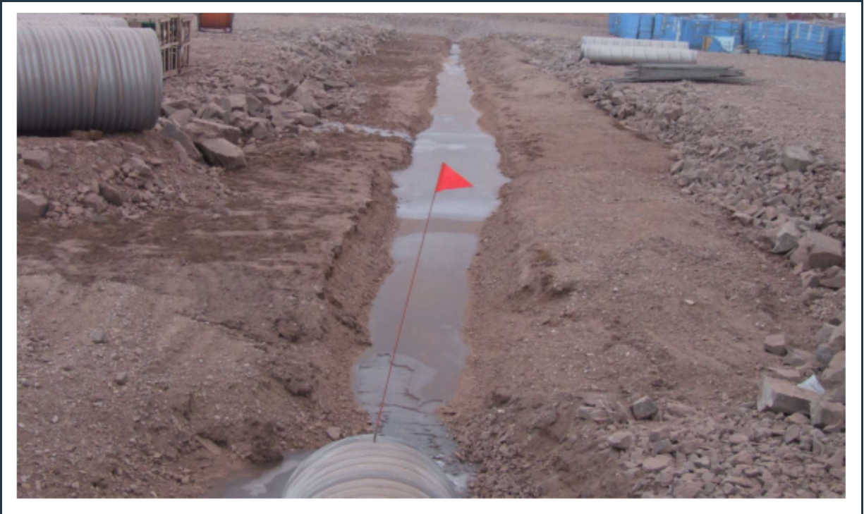
Figure 57: W3-W14 surface water collection ditch (still under construction).
