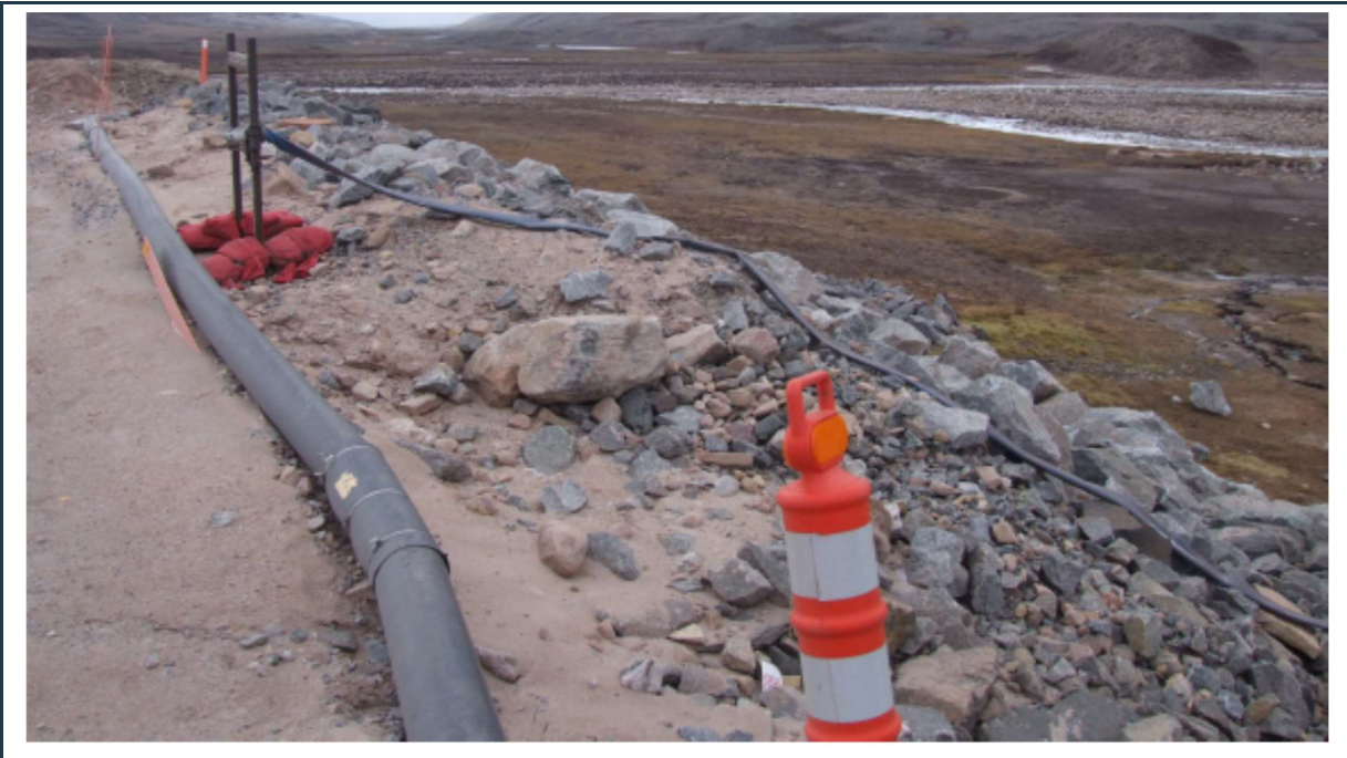
Figure 37: Water (effluent) discharge area. Stable slope, comprising a mix of crushed rock and soils.
