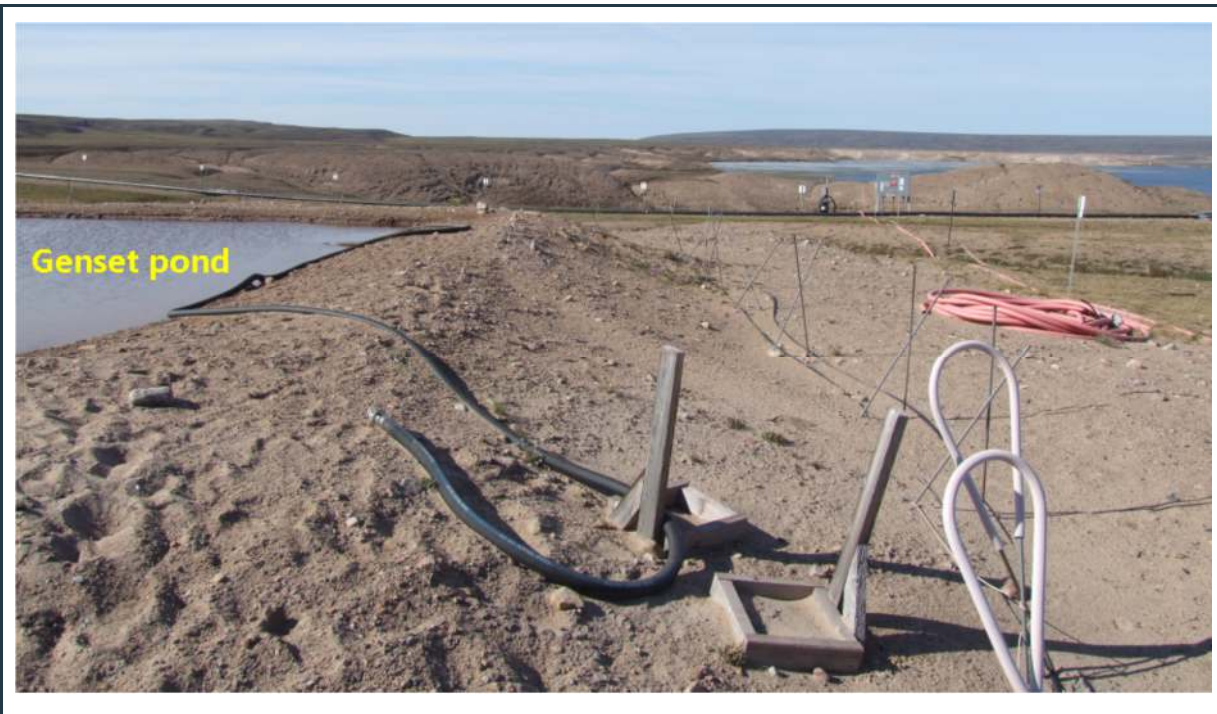
Figure 29: View of the berm at the Genset pond
