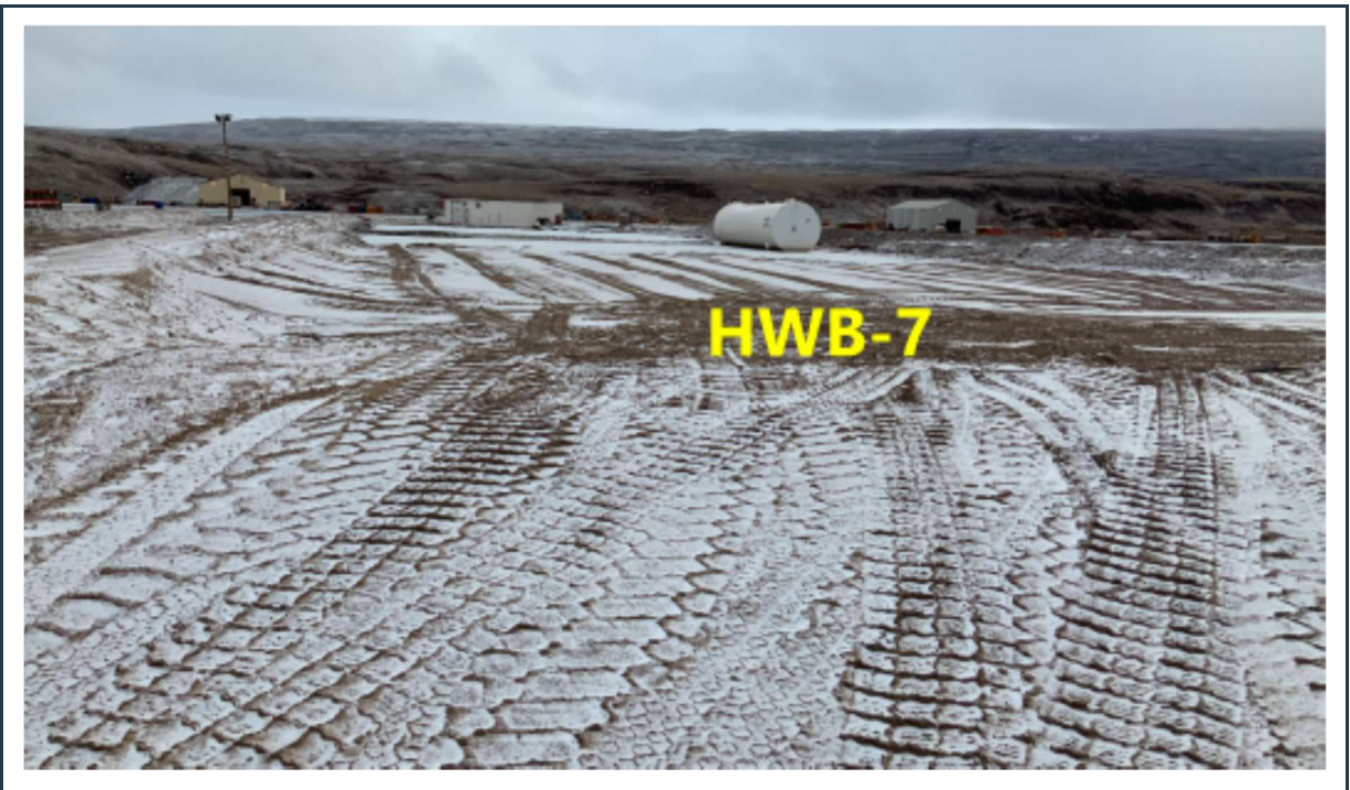
Figure 16: View of HWB-7, with only one fuel tank stored in the large cell.
