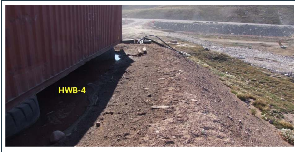
Figure 46: Stable berm at the HWB-4 pond
