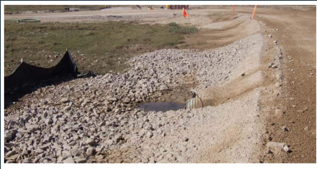
Figure 102: View of culvert 202 (outlet)
