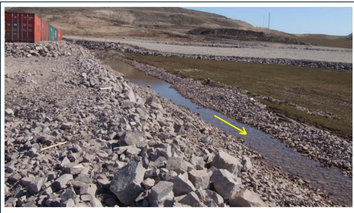
Figure 67: 380 M surface water collection ditch (under construction)
