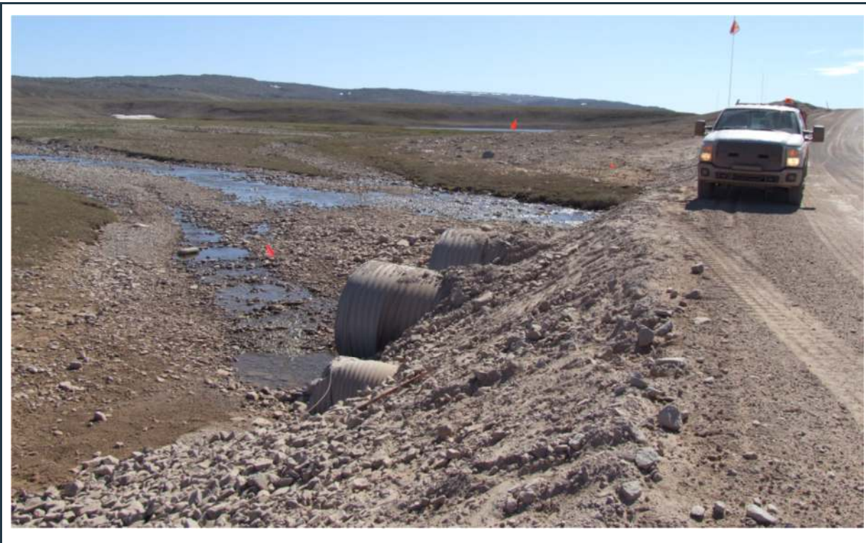
Figure 85: View of culvert(s) 078 (inlet)
