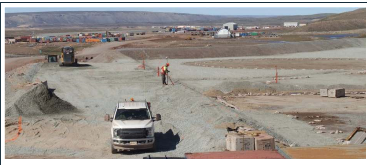
Figure 35: View of the new fuel tank farm (under construction)
