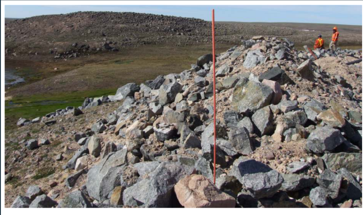
Figure 40: Water discharge area. Stable slope, comprising a mix of crushed rock and soils.
