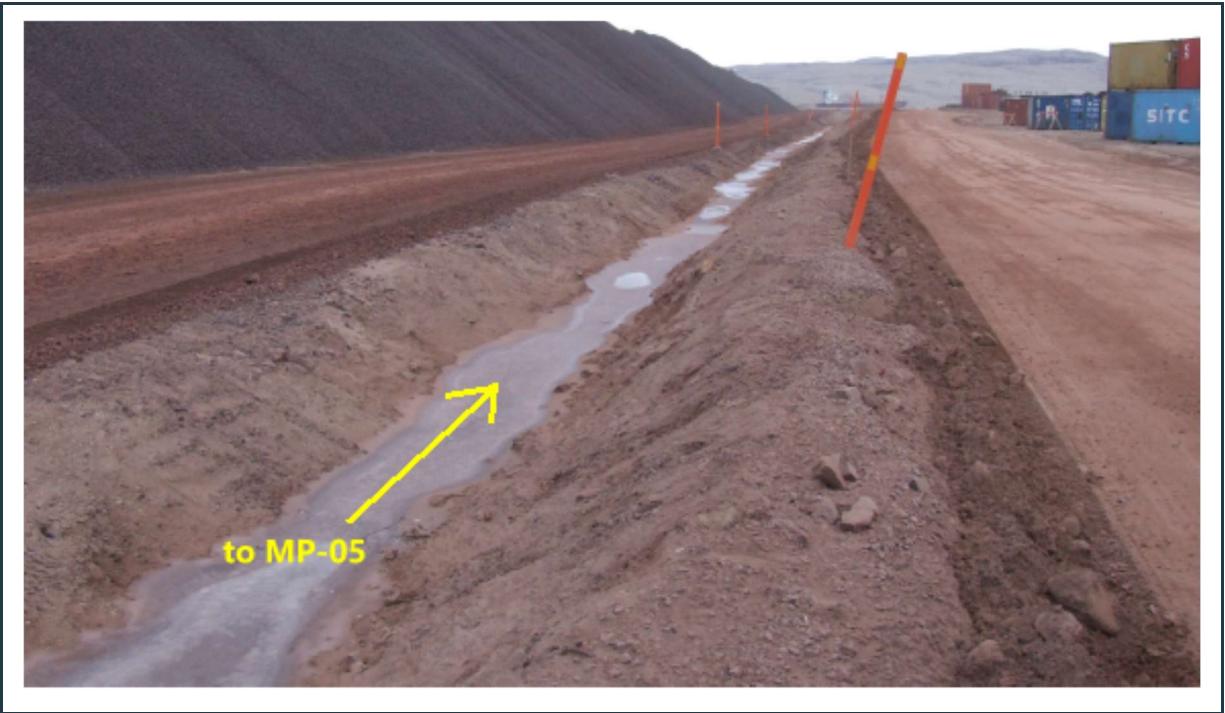
Figure 51: Surface water collection ditch, adjacent to the ore stockpile (leading to the MP-05 pond).
