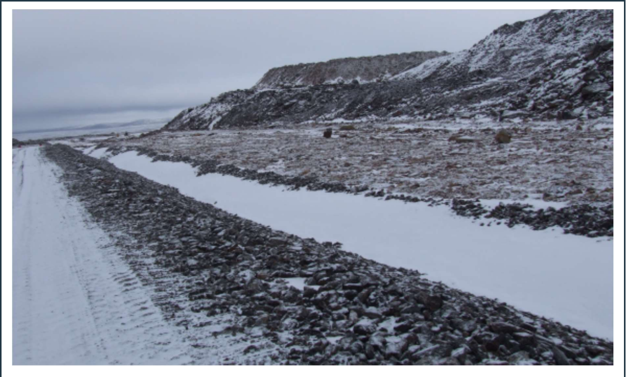
Figure 23: Snow-filled ditch under construction around the waste rock dump (north-west side).
