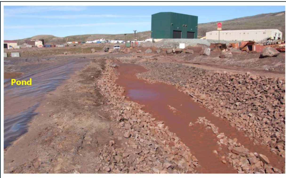
Figure 23: MS-06 surface water collection pond and side-ditch
