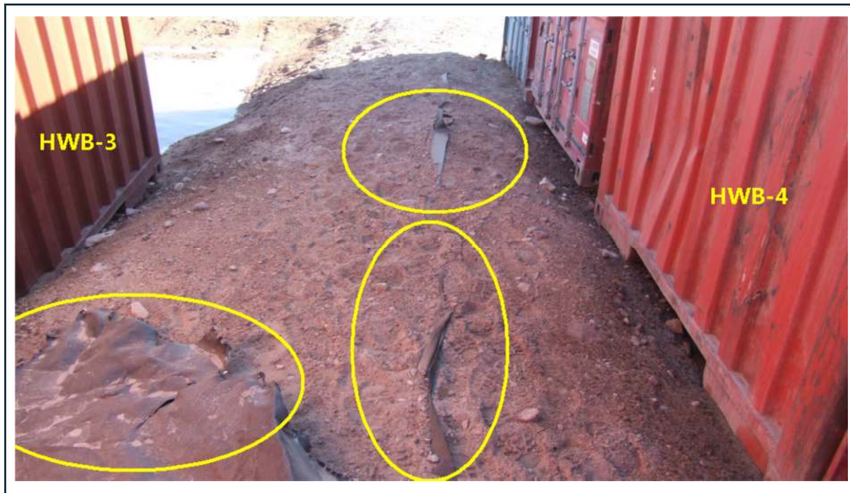
Figure 47: Exposed liner between the HWB 3 and HWB-4 ponds
