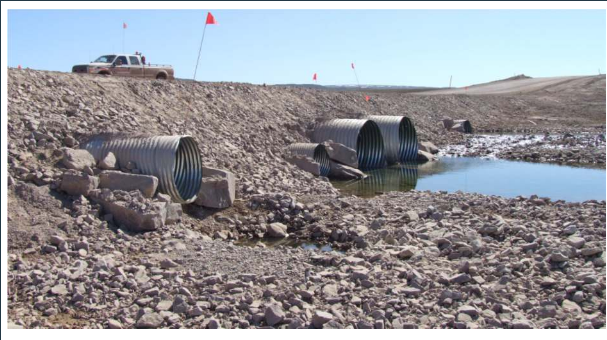
Figure 84: View of culvert(s) 078 (outlet)
