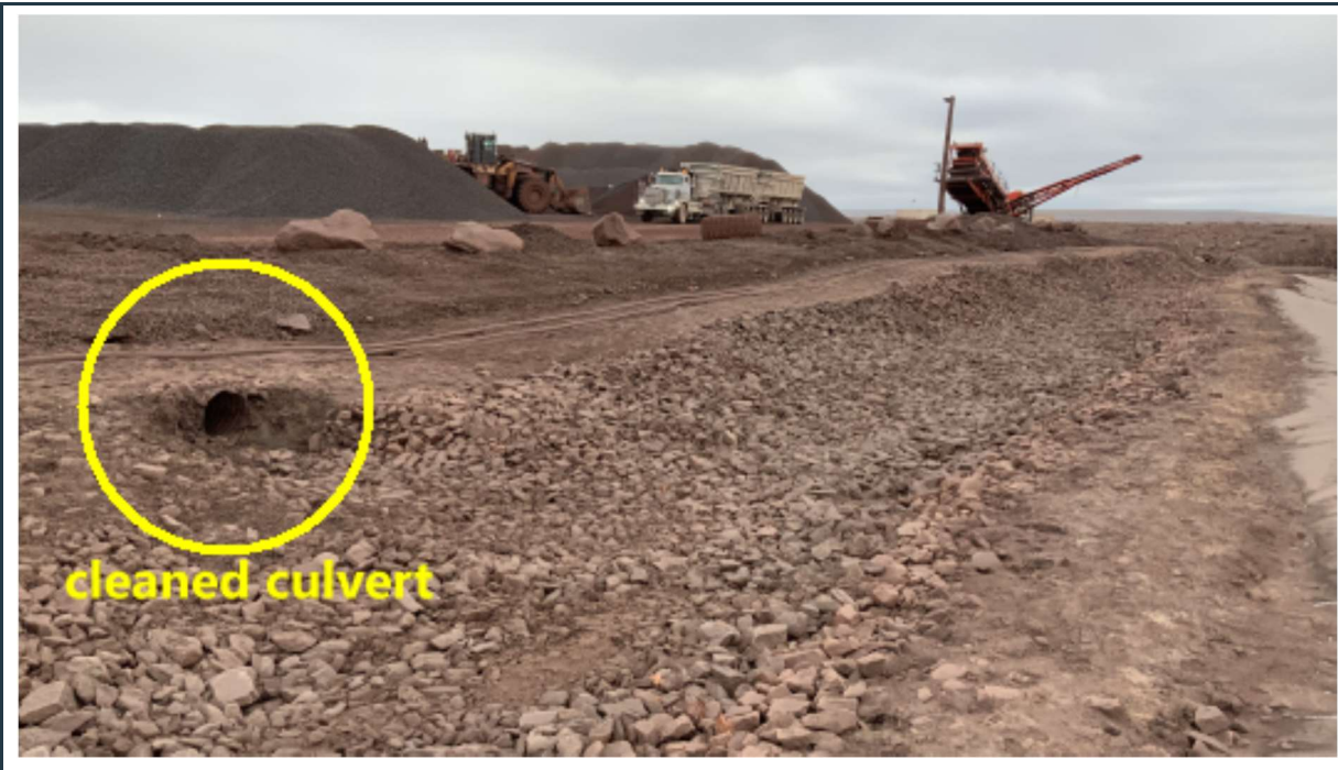
Figure 19: Surface water collection ditch, with recently cleaned culvert.
