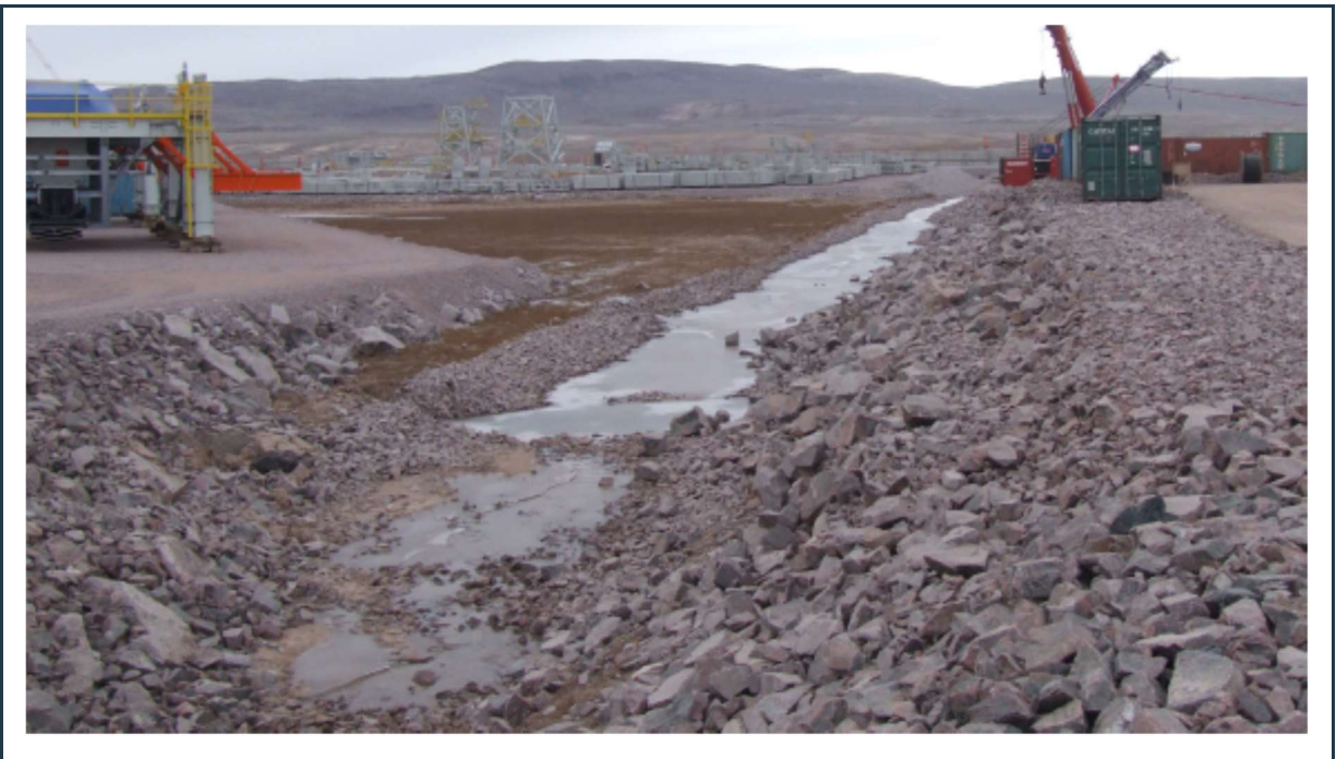
Figure 58: "380 M" surface water collection ditch (under construction).
