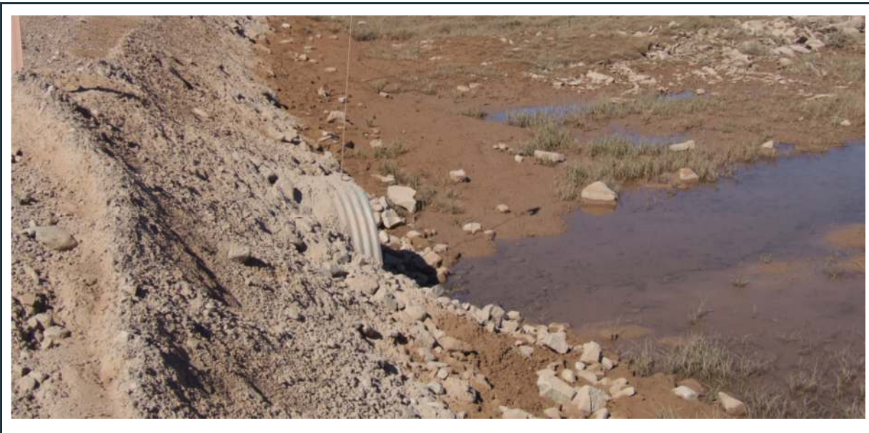
Figure 83: View of culvert 076 (inlet)
