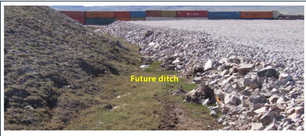
Figure 62: Future “P-SWD-3 LP2” surface water collection ditch – under construction
