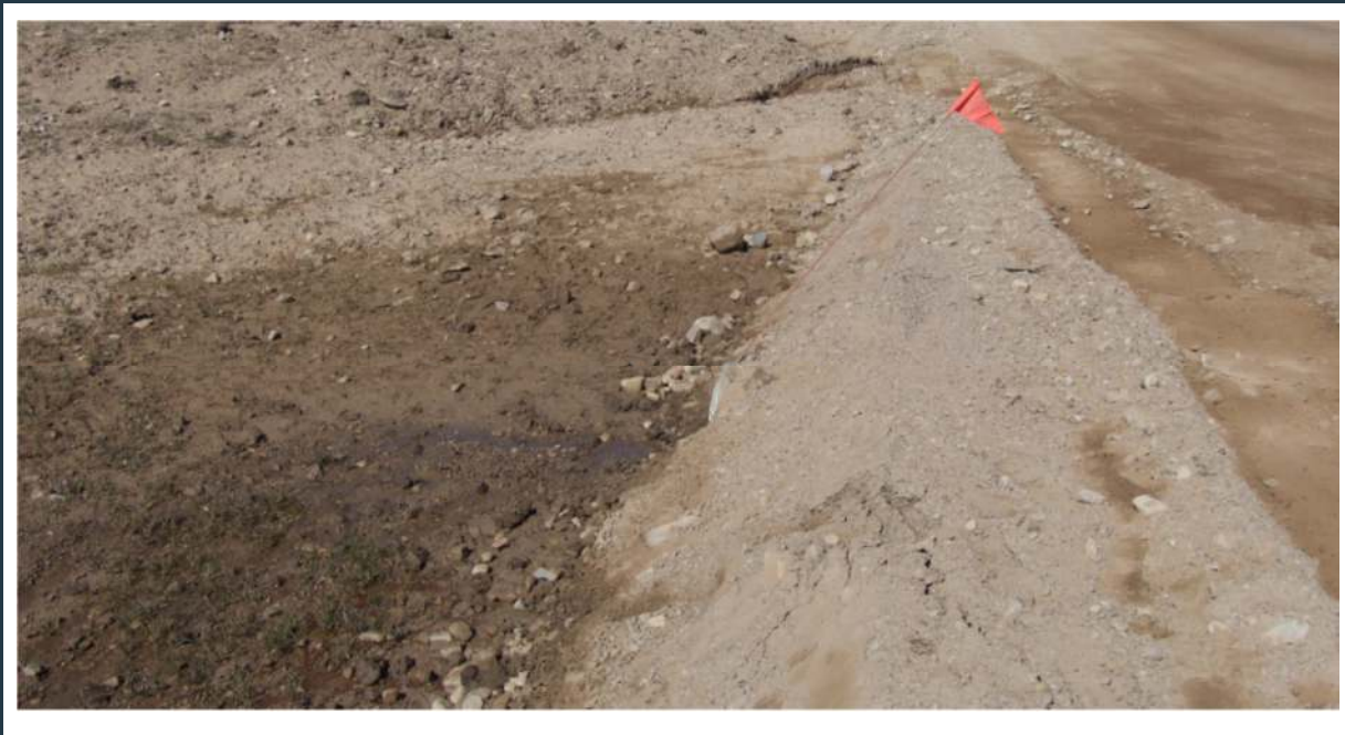
Figure 92: View of culvert 107 (outlet)
