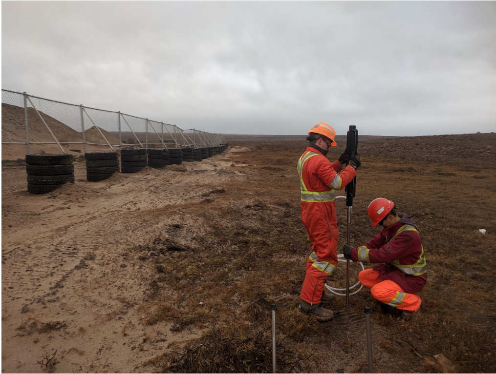
Figure 2: Installation of MS-LF-GW1 on September 27, 2019
