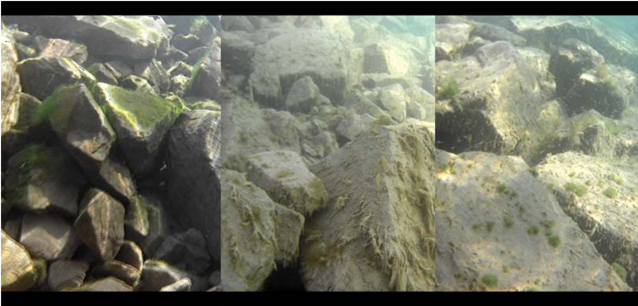
Figure 3: Armour stone around ore dock – still images from underwater video collected in 2017.
