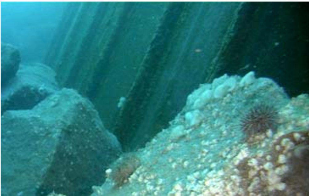
Figure 6: Barnacles and urchins observed on armour stone along east side of ore dock in 2017.
