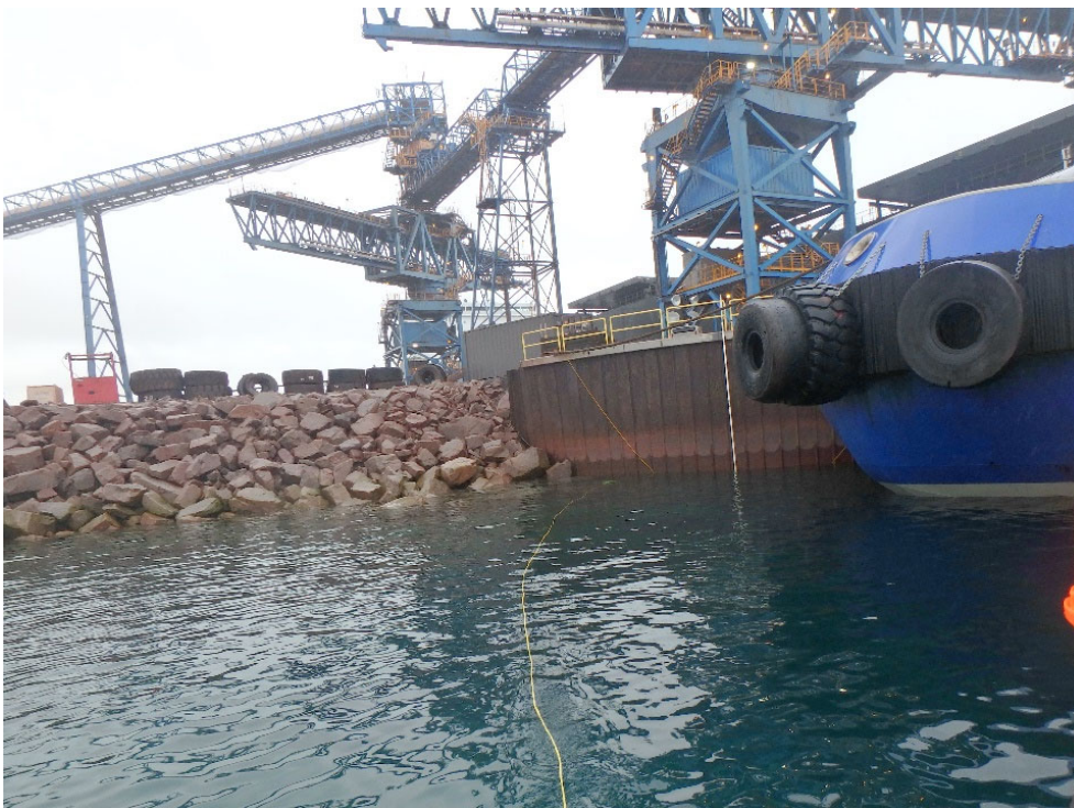
Photo 2: Topside view of underwater video survey of offset habitat along Transect 7 (T7) on east side of Milne Port Ore Dock in August 2019
