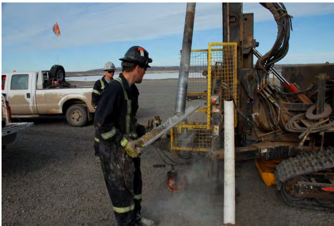
PHOTO 8 – Geotechnical Investigation at Hole 1, June 2017
