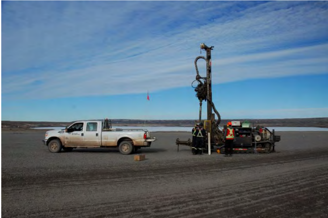
PHOTO 3 - Pre-Drilling Site Conditions at Hole 1, June 2017
