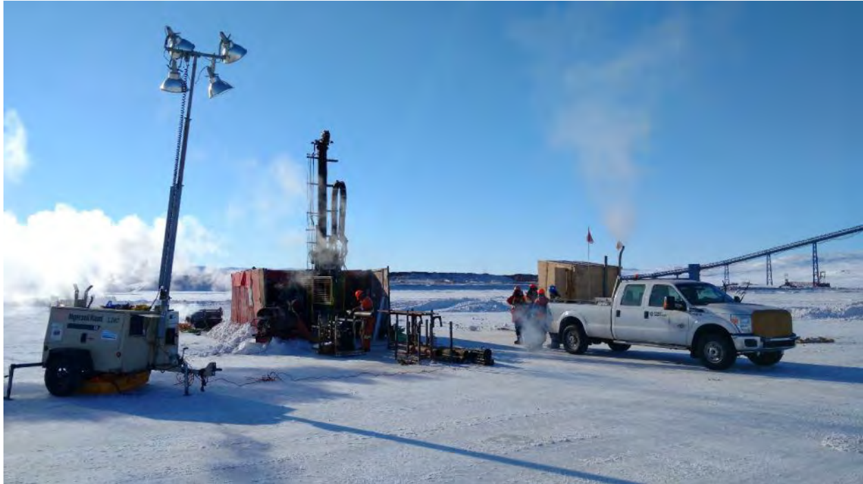
PHOTO 1 - Geotechnical Drilling Operations at BH17-D005, March 2017
