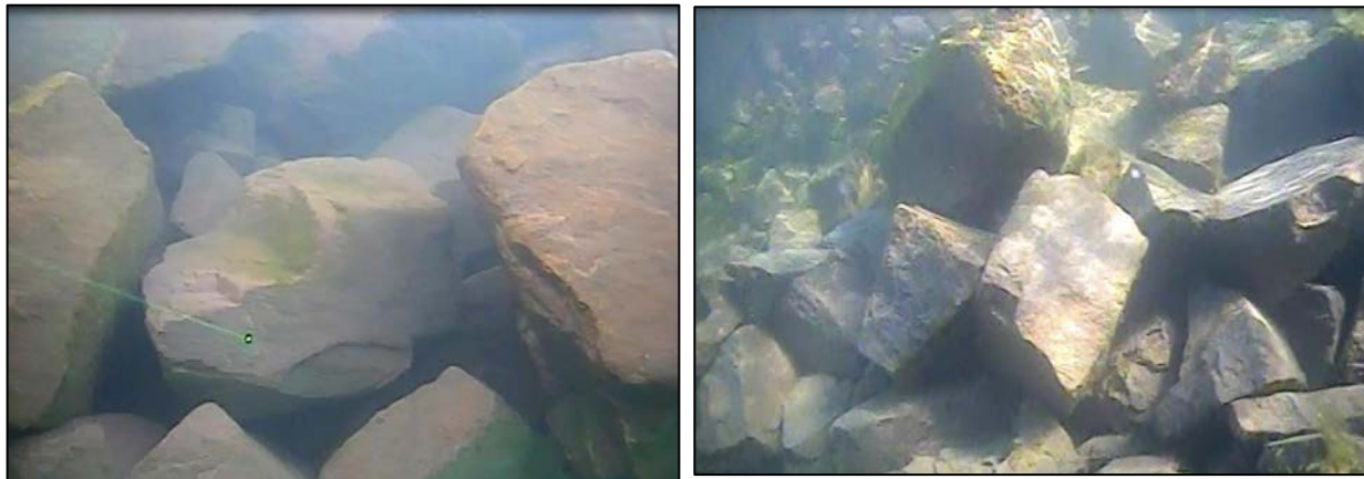
Figure 10 Screen Captures for Video Documenting the Stability of Armour Stone at the Milne Ore Dock, 2016.
