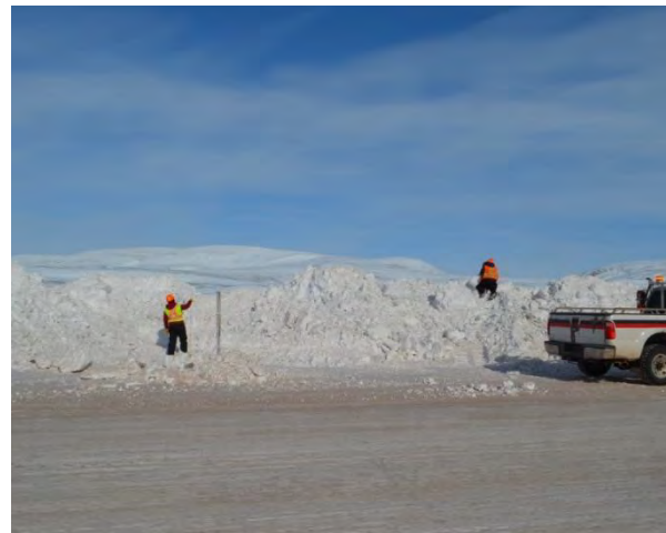
Photo 14 Example of snow bank conditions >2 m at km 16 on the Tote Road, April 21, 2017.
