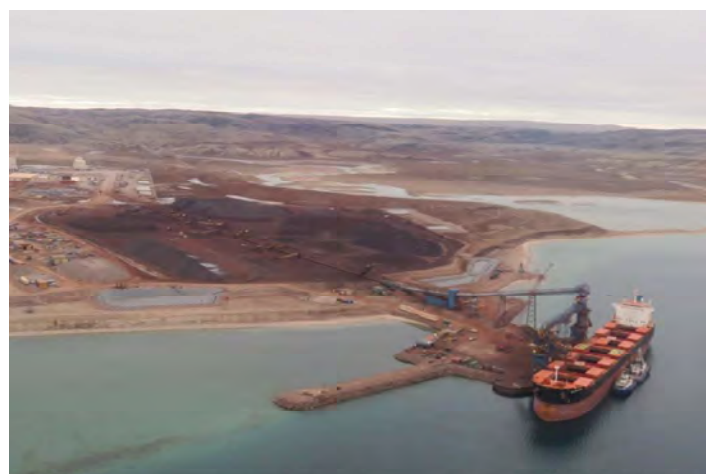
Vessel Being Loaded with Iron Ore at the Milne Port using Ship Loading Conveyors
