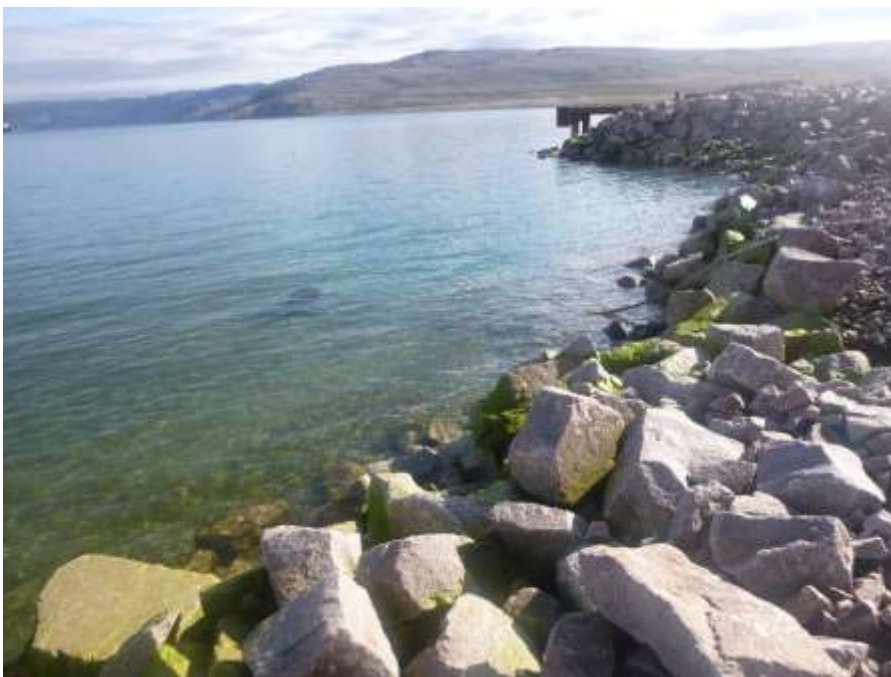
Photo 2: North side of Freight Dock, looking northeast during site visit on 7 August 2020 at 0.4 m tide. Water depth approx. -1.0 to -1.2 m CD. Green filamentous algae observed on the sides/edges of riprap substrate within intertidal/upper subtidal depth contours.
