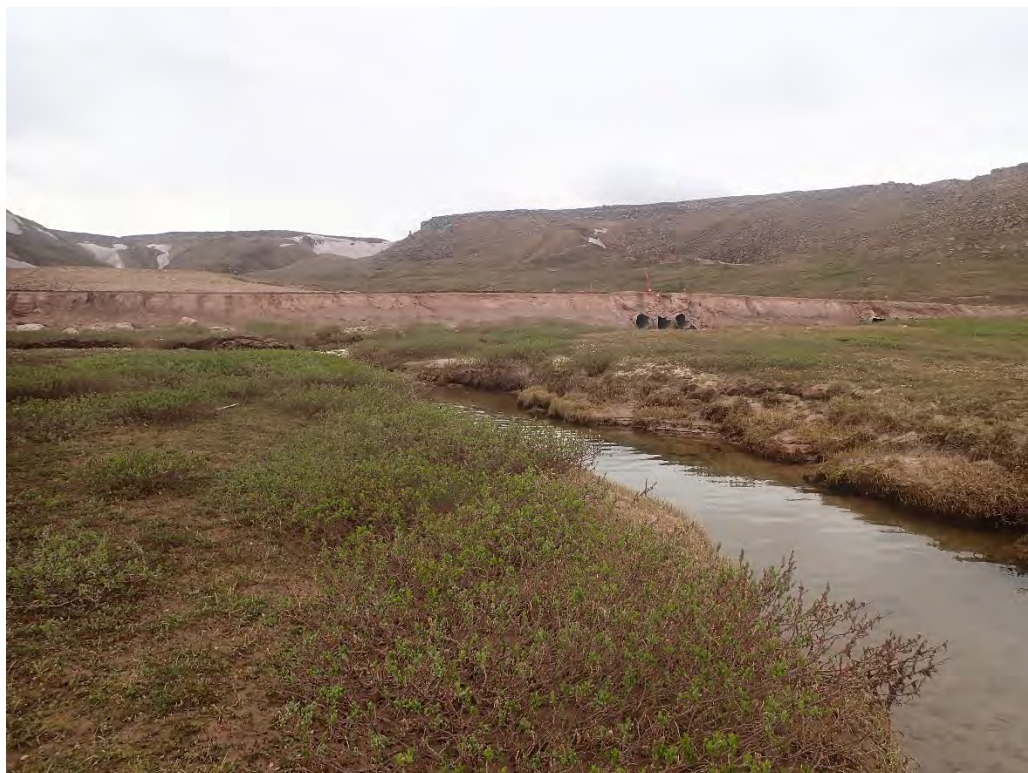
Photo 4. BG-24 Culvert Crossing Downstream on July 05, 2021
