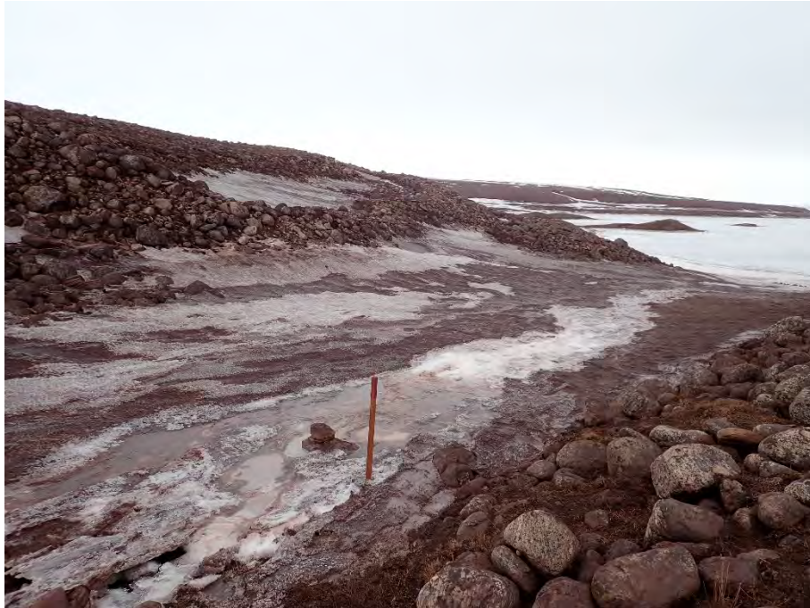
Photo 1. LDFG Outfall on May 6, 2021
