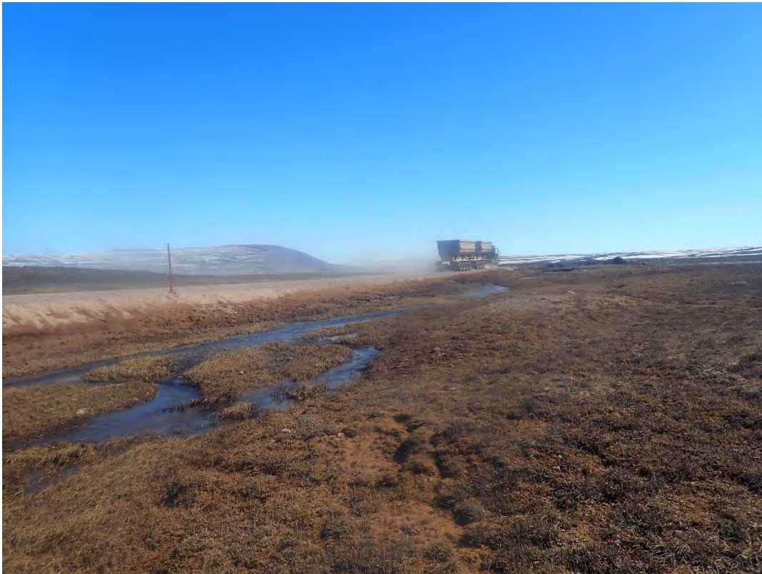
Photo 4. CV-001 Culvert Crossing Downstream on June 8, 2021
