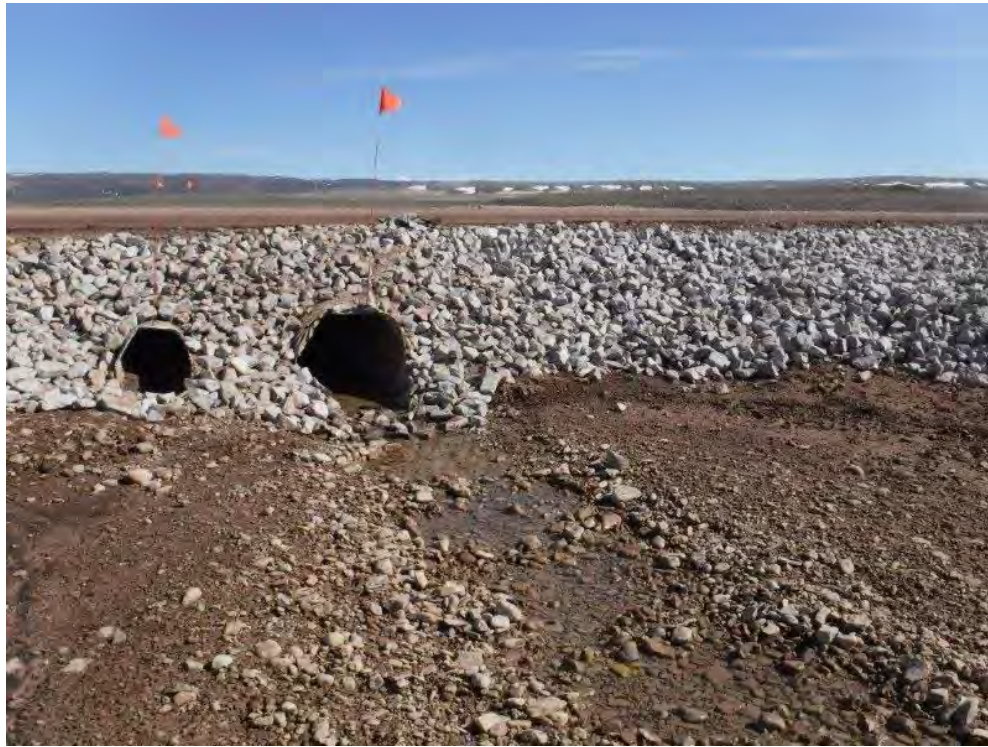
Photo 5. CV-115 Culvert Crossing Downstream July 9 2021
