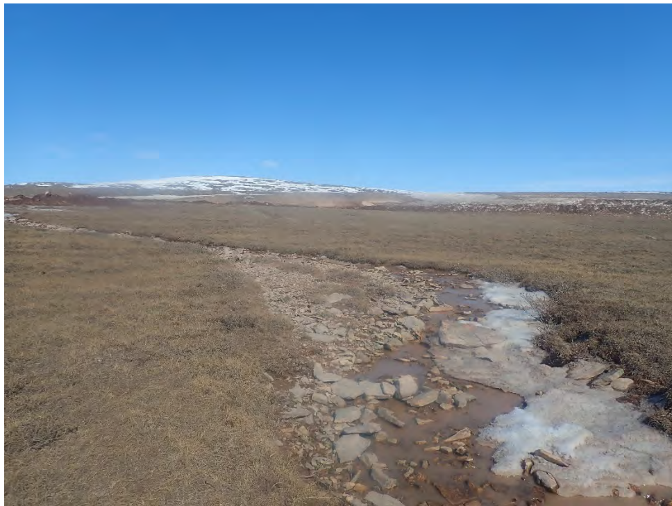
Photo 2. CV-112 Culvert Crossing Downstream on June 1, 2021
