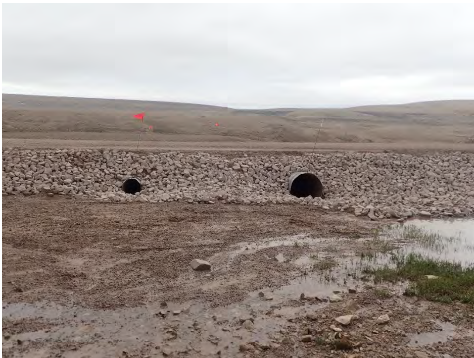
Photo 4. CV-093 Culvert Crossing Upstream July 13 2021
