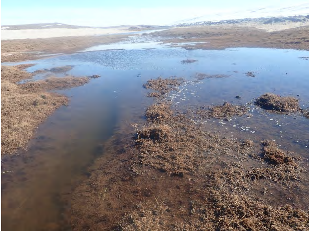
Photo 1. CV-115 Culvert Crossing Upstream on June 1, 2021
