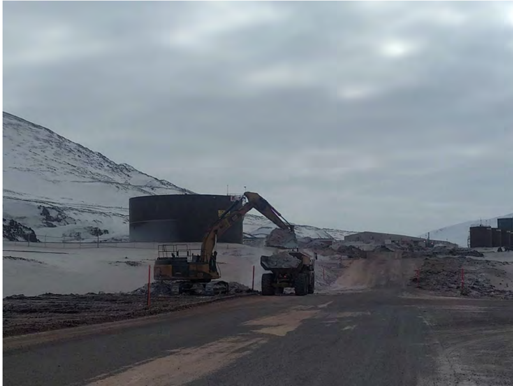
Photo 1. Snow Removal CV-186 to CV-187 Upstream of SDLT-OUT on April 20, 2021
