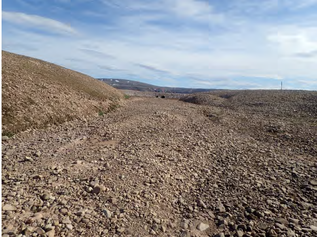
Photo 6. CV-115 Culvert Crossing Downstream July 11 2021
