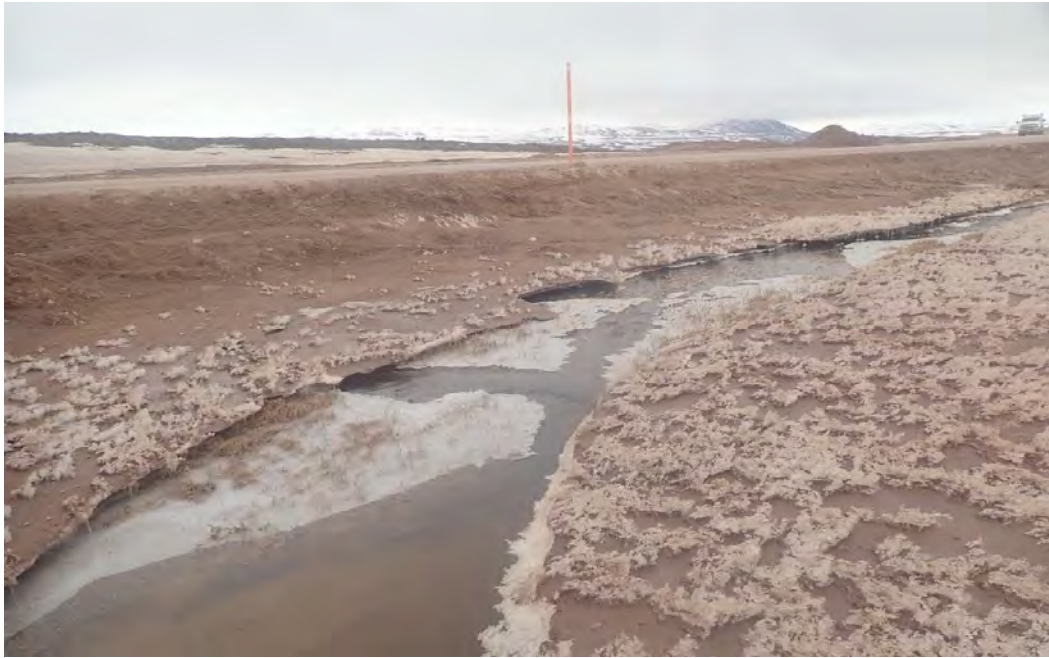
Photo 3. CV-001 Culvert Crossing Downstream on May 31, 2021
