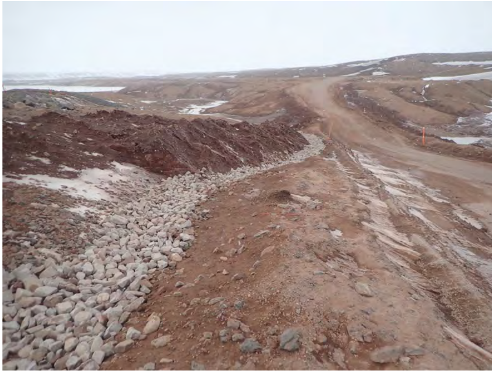
Photo 3. BG-01 Downstream Ditch Riprap Armouring (May 13, 2021)
