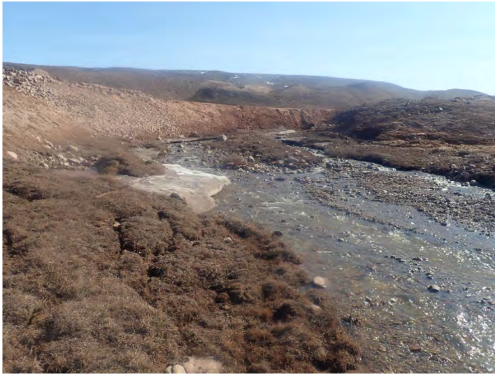
Photo 3. CV-154-A Culvert Crossing Downstream on June 10, 2021
