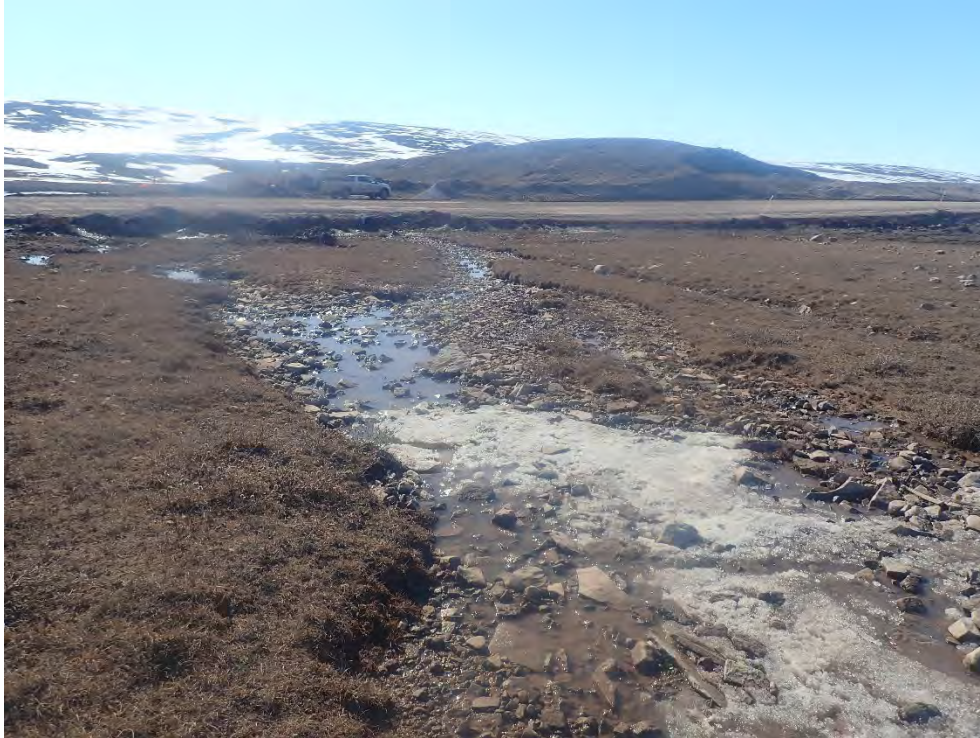
Photo 1. CV-112 Culvert Crossing Upstream on June 1, 2021
