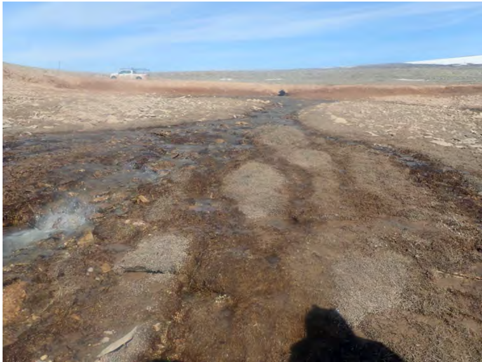
Photo 3. CV-093 Culvert Crossing Downstream on June 14, 2021
