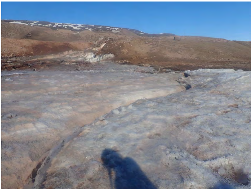
Photo 2. CV-154-A Culvert Crossing Downstream on June 1, 2021
