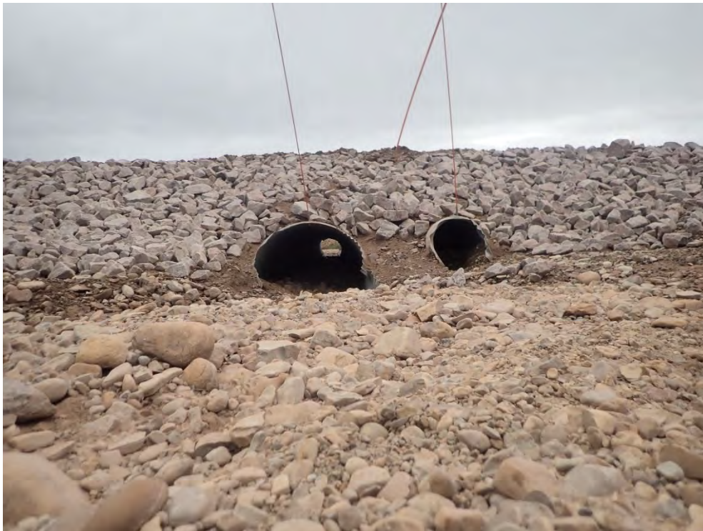
Photo 4. CV-115 Culvert Crossing Upstream July 9 2021
