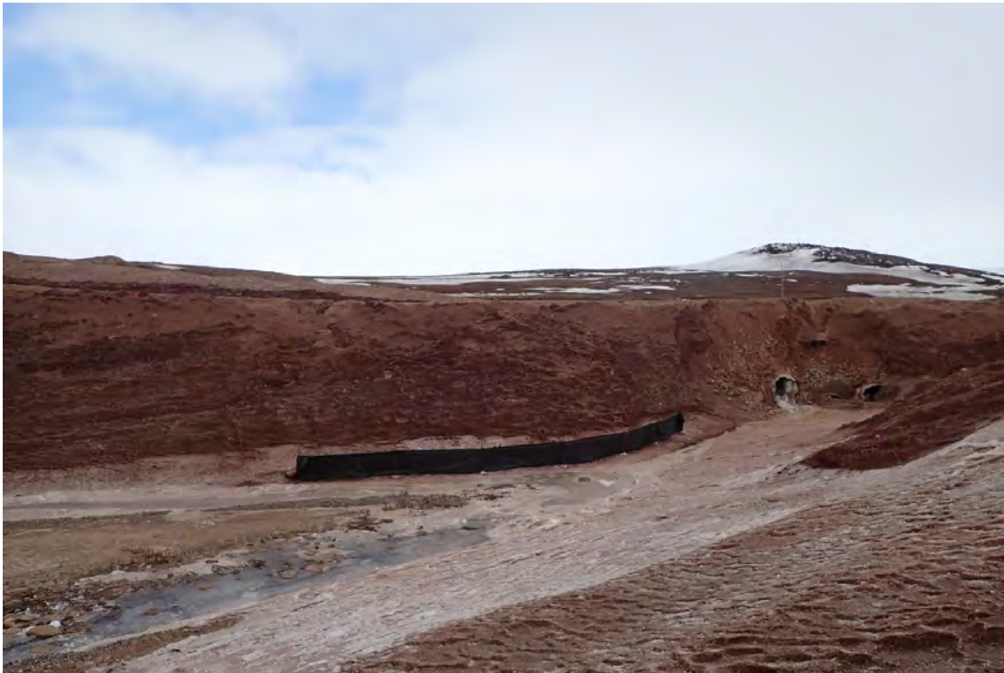
Photo 4. Silt Fencing at the Outlet of BG-01 (May 15, 2021)
