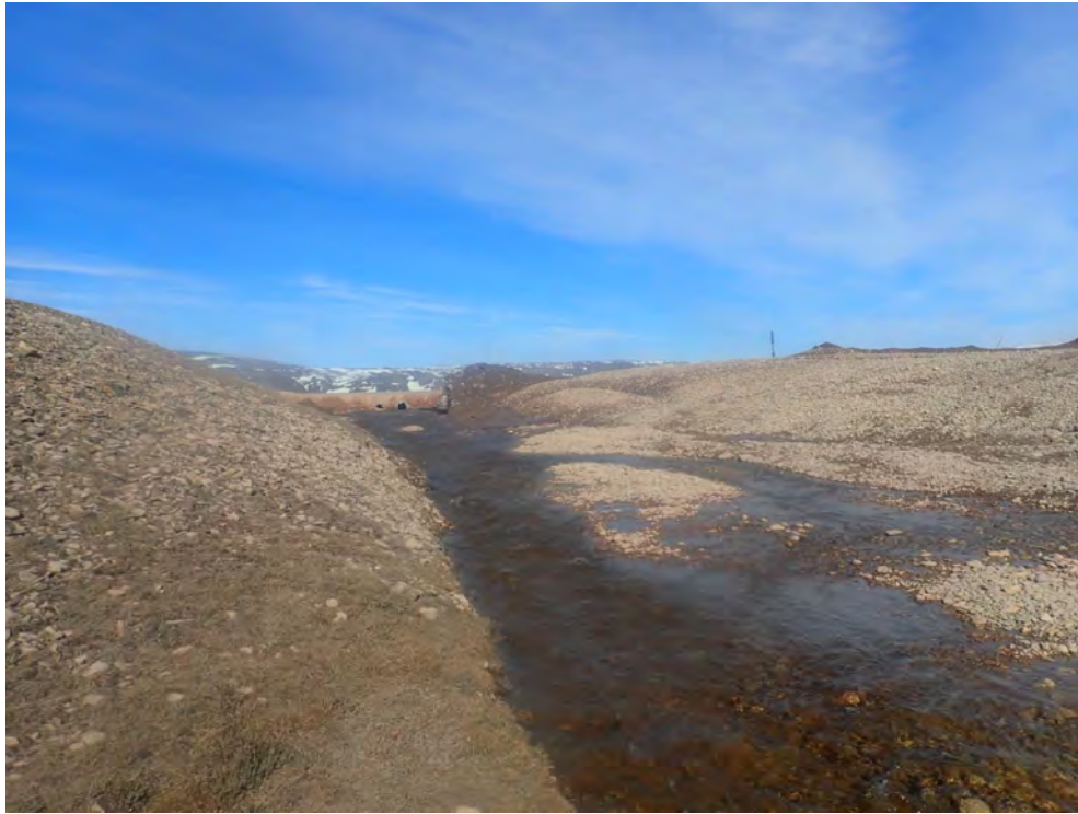
Photo 3. CV-115 Culvert Crossing Downstream on June 9, 2021
