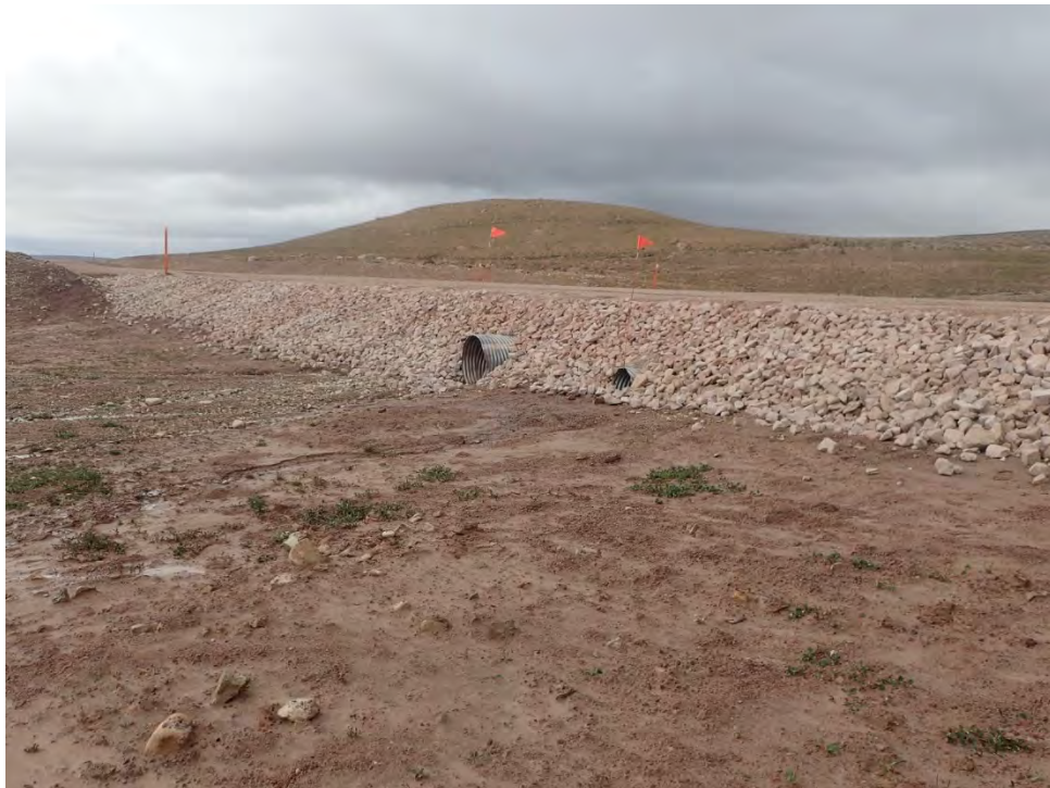
Photo 5. CV-093 Culvert Crossing Downstream July 13 2021
