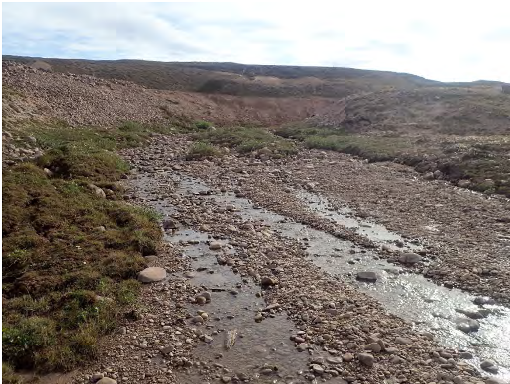
Photo 4. CV-154-A Culvert Crossing Downstream on July 11, 2021
