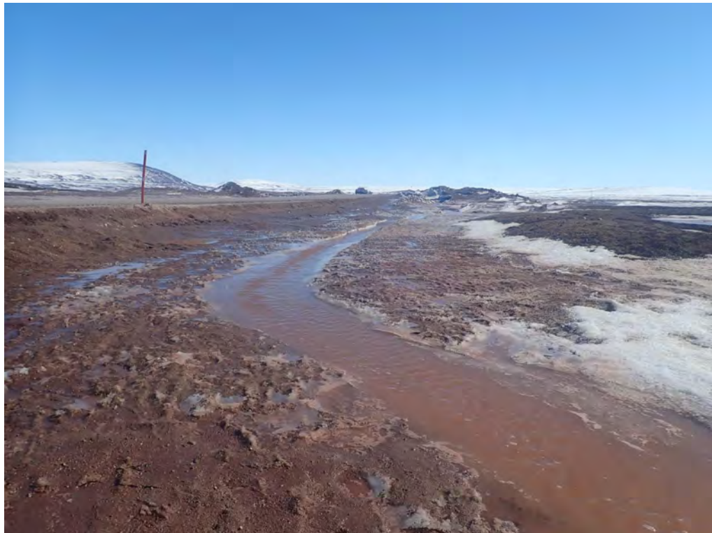
Photo 2. CV-001 Culvert Crossing Downstream on May 26, 2021
