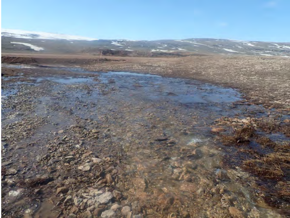
Photo 1. CV-093 Culvert Crossing Upstream on June 9, 2021
