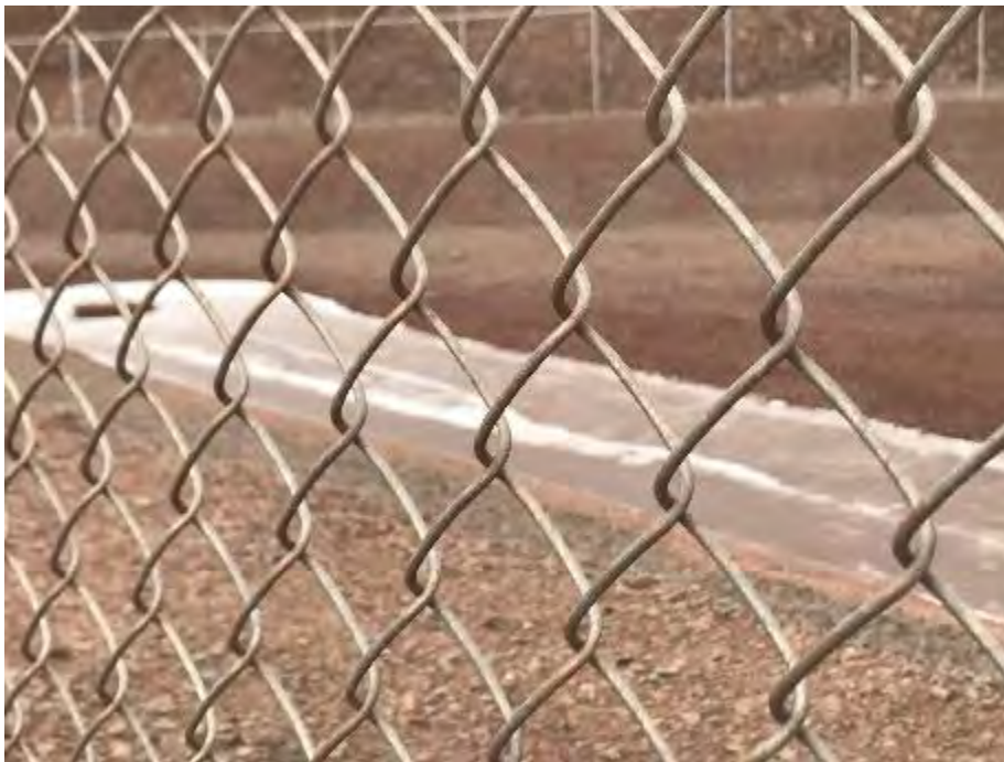
Photo 49: Site Reconnaissance at Fuel Farm MS03. September 27, 2021
