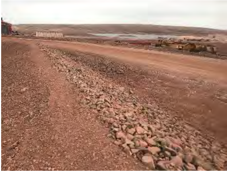
Photo 56: Site Reconnaissance at Fuel Farm MS03B, facing west. September 27, 2021
