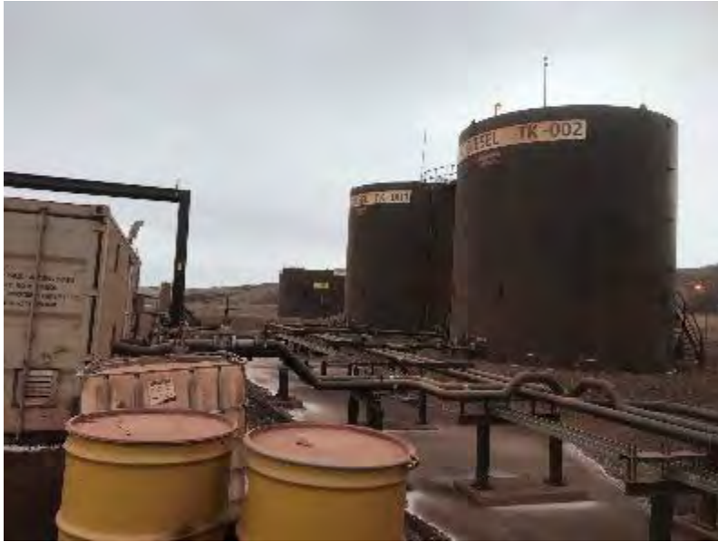
Photo 52: Site Reconnaissance at Fuel Farm MS03B. September 27, 2021
