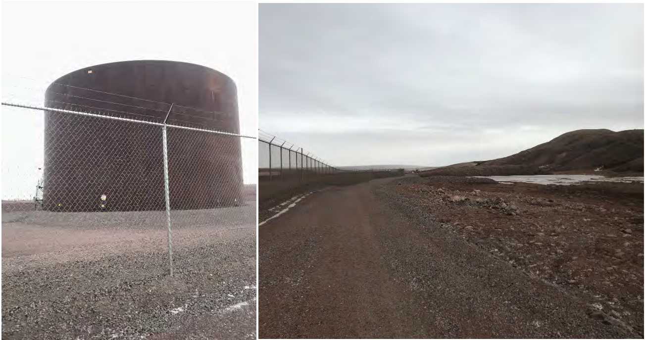
Photo 48: Site Reconnaissance at Fuel Farm MS03. September 27, 2021
