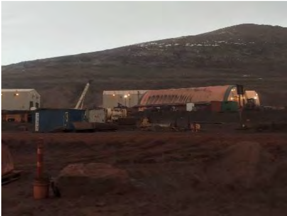
Photo 45: Site Reconnaissance at Crusher Area Berm, facing northwest. September 27, 2021
