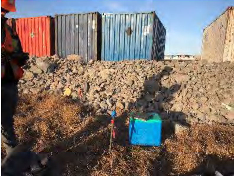
Photo 36: Monitoring location MS-HWB-GW-REF1, facing west. September 26, 2021
