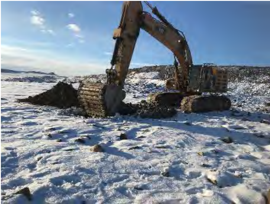
Photo 15: Site Reconnaissance: MS-WRF-TP1. September 25, 2021
