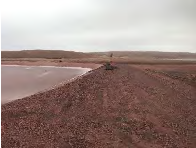
Photo 44: Site Reconnaissance at Crusher Area Berm, facing south. September 27, 2021
