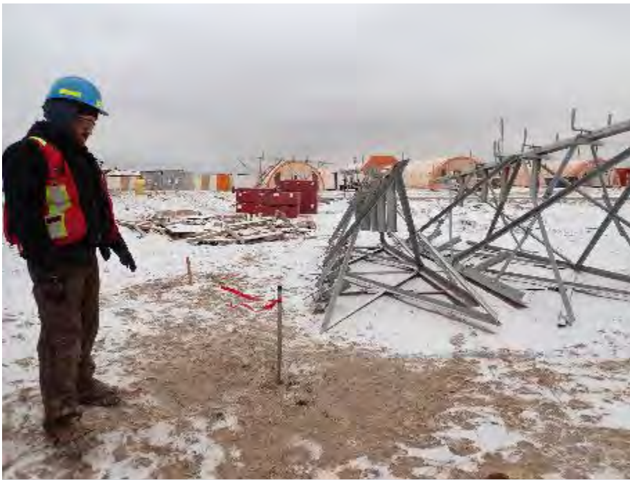
Photo 4: Drive-point piezometer installation - monitoring location MS-HWB-GW5, facing south. September 19, 2021
