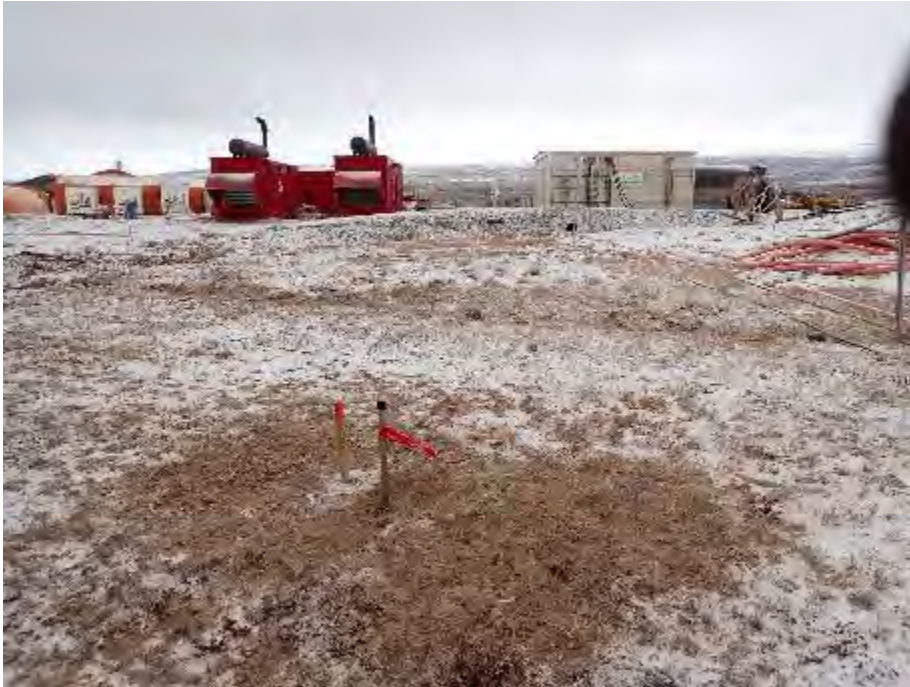
Photo 5: Drive-point piezometer installation - monitoring location MS-HWB-GW6, facing west. September 19, 2021
