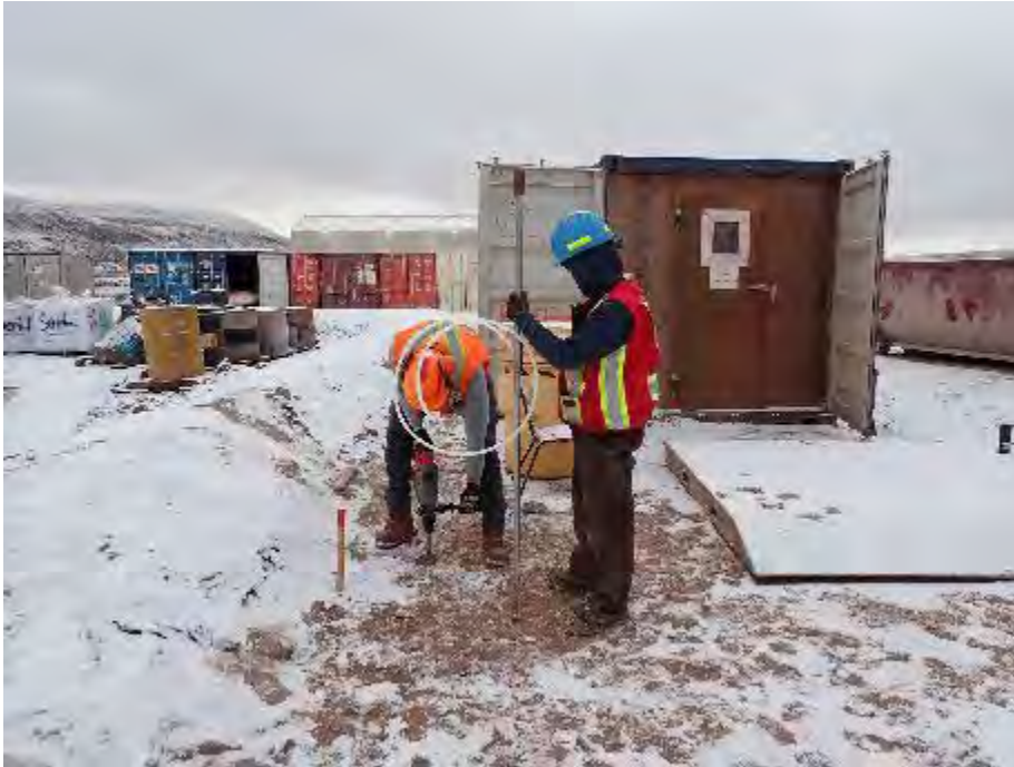
Photo 1: Drive-point piezometer installation - monitoring location MS-HWB-GW2, facing east . September 19, 2021
