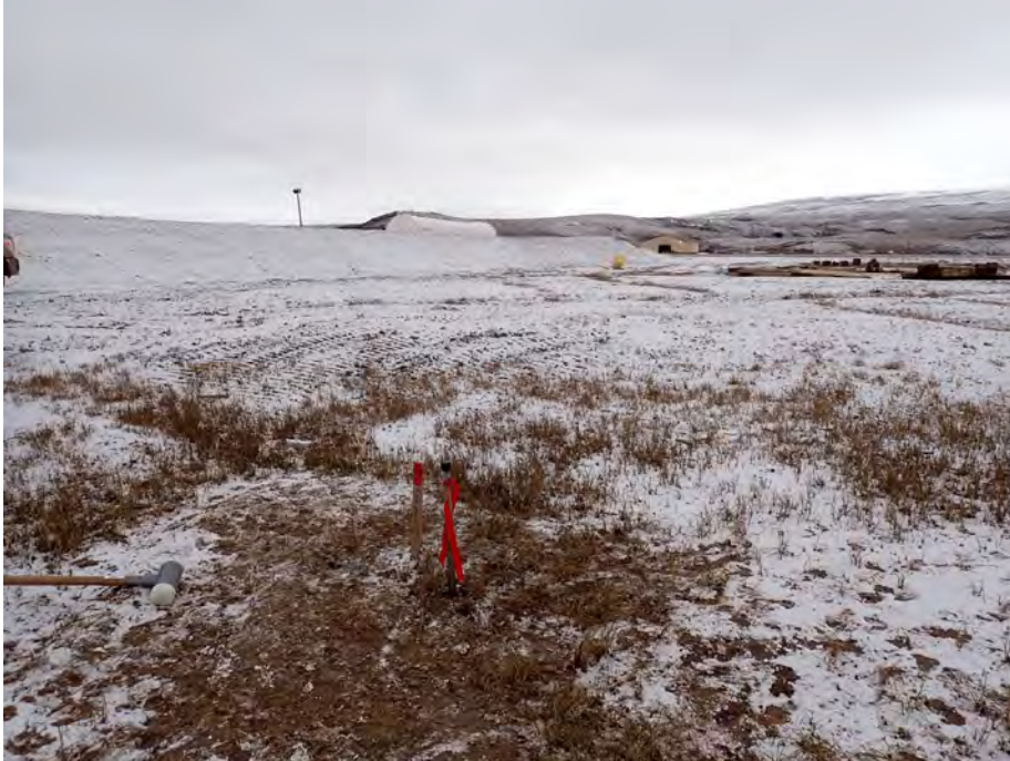
Photo 7: Drive-point piezometer installation - monitoring location MS-HWB-GW-REF3, facing northwest. September 19, 2021
