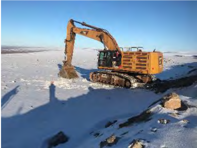
Photo 20: Site Reconnaissance: MS-WRF-TP2. September 25, 2021
