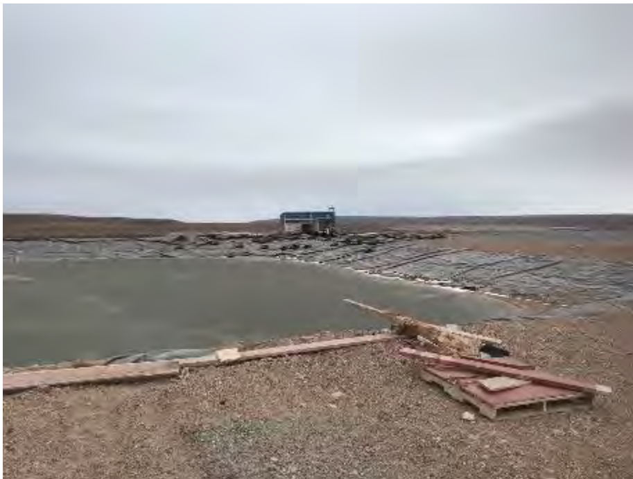
Photo 59: Site Reconnaissance at PWSP Polishing Waste Settling Ponds, facing west. September 27, 2021
