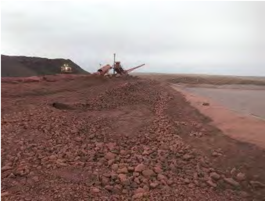
Photo 43: Site Reconnaissance at Crusher Area Berm, facing east. September 27, 2021
