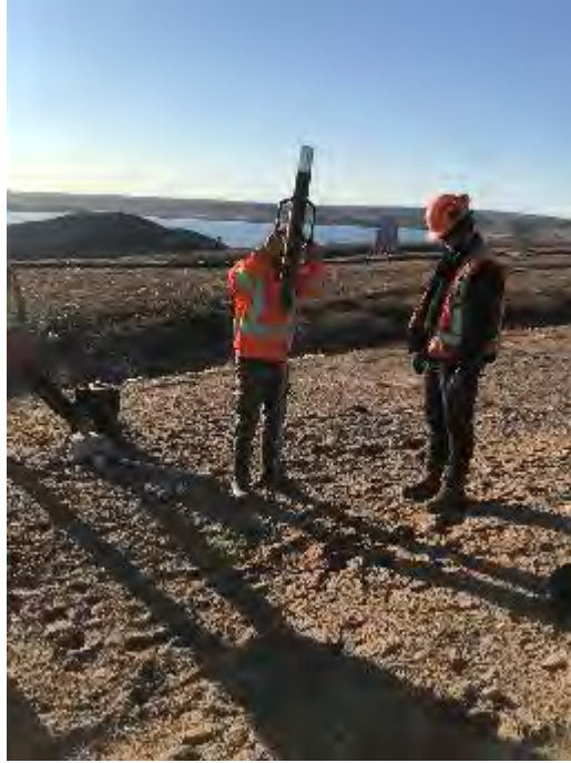
Photo 10: Installation of drive-point piezometer at monitoring location MS-HWB-GW8, facing southeast. September 22, 2021
