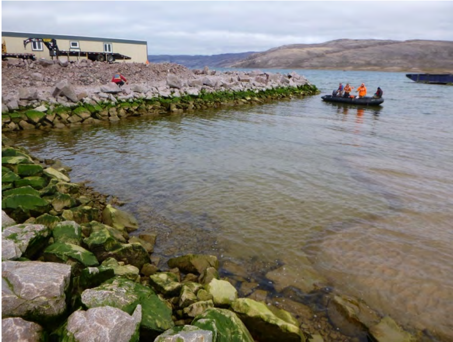
Photo 1: East side of Freight Dock (facing northeast) during site visit on 18 August 2021 at 0.7 m tide. Green filamentous macroalgae observed on coarse rock substrate in intertidal zone.
