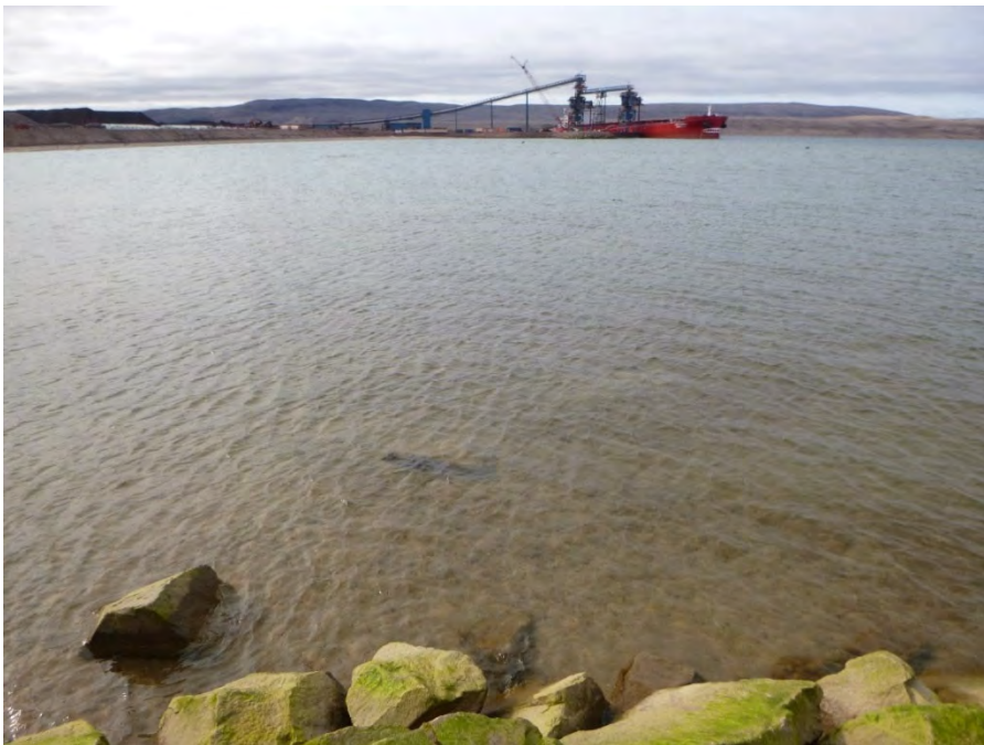
Photo 8: West side of Freight Dock (facing west towards Ore Dock) during site visit on 18 August 2021 at 0.7 m tide.
