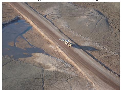
Photo 21: 740 Tire Drag for Dust Suppression – September 2019
