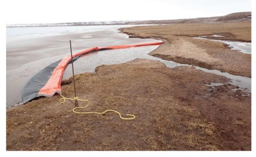
Photo 24: Silt Curtain Installation at Camp Lake Settling Ponds - May 2019
