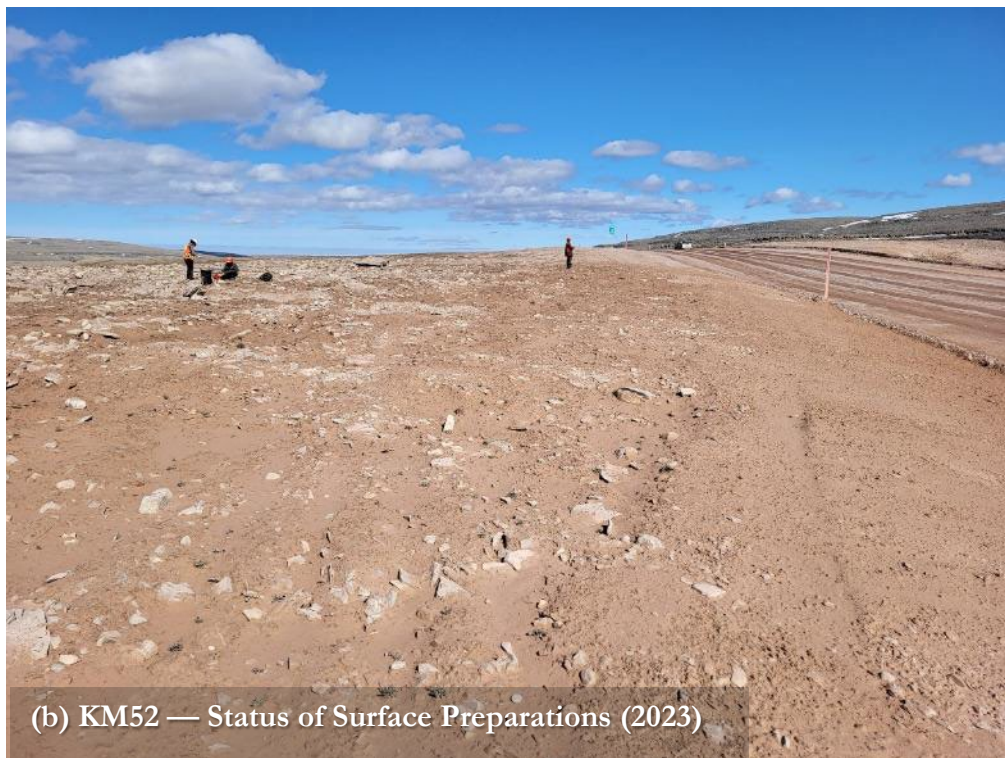
Photo 20. KM52 — 2023 Status of Cover Vegetation (a) and Surface Preparations (b).
