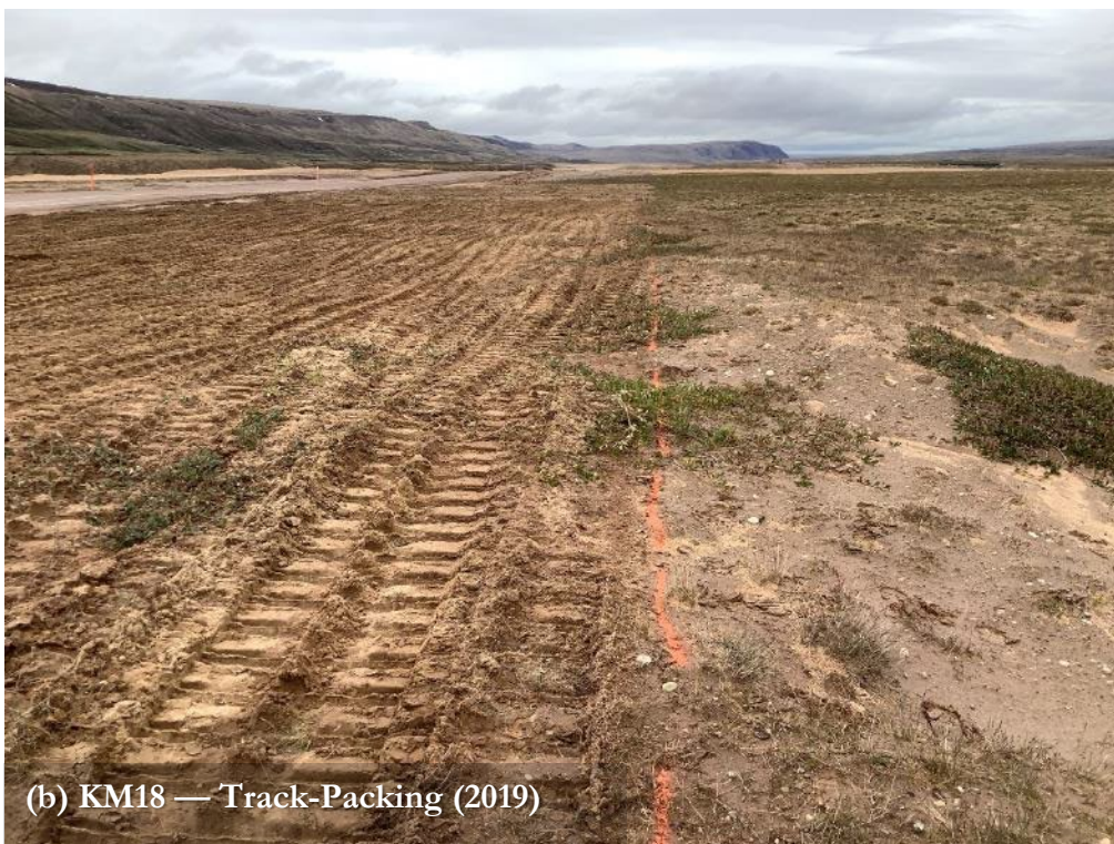
Photo 12. KM18 — Initial site preparation (a) and surface track-packing (b).
