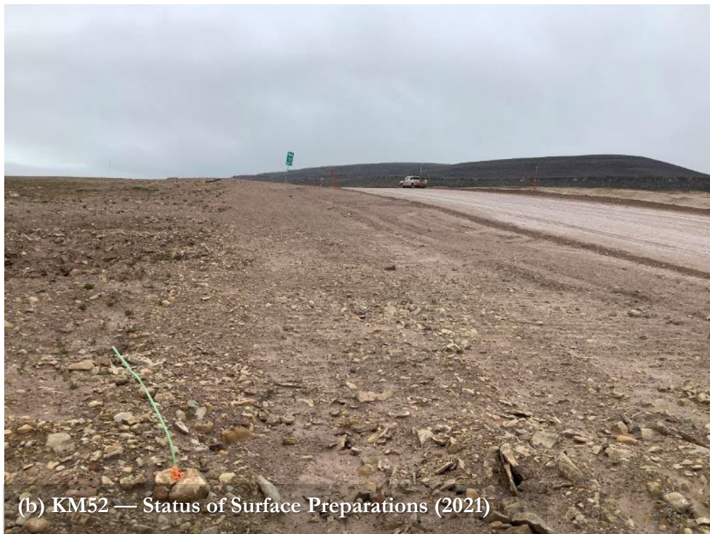
Photo 14. KM52 — 2021 Status of Cover Vegetation (a) and Surface Preparations (b).
