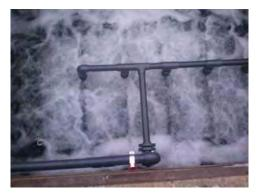
Proper air scouring in membrane tank
